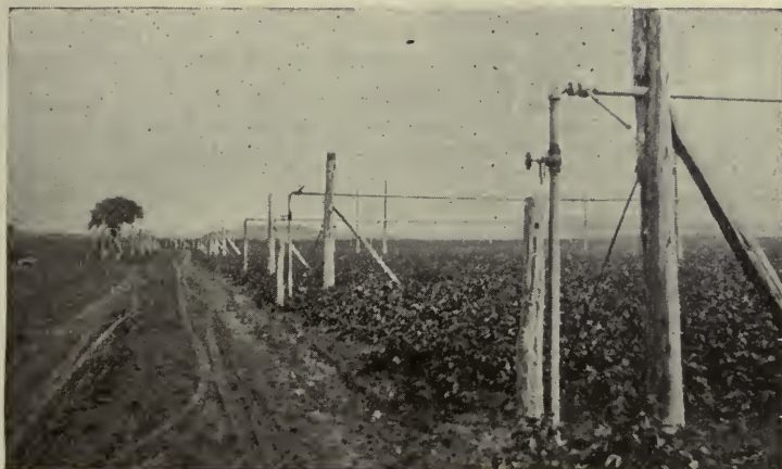
FIG. 106.—Intensive potato culture on a Long Island farm, under the "Skinner system" of irrigation.
