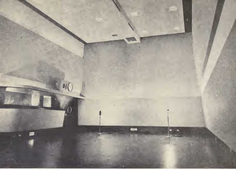
Figure 7. Live-end dead-end studio with slanting walls.
