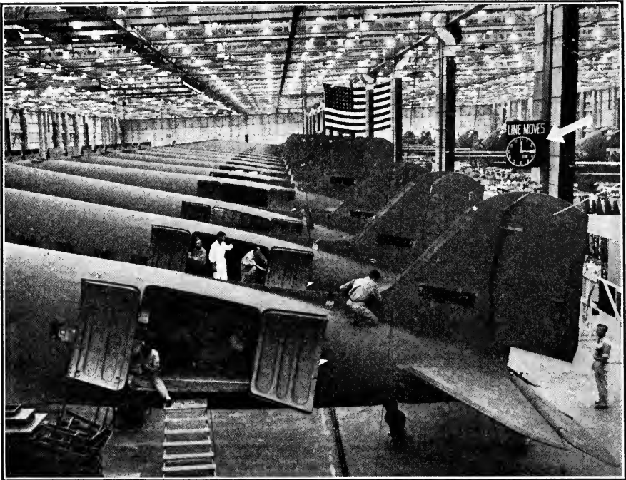
FIG. 57.—The hands on the clock face are set to indicate when the line will next move. Here is intermittent movement and a long cycle time. (Courtesy of Douglas Aircraft Company, Inc.)
