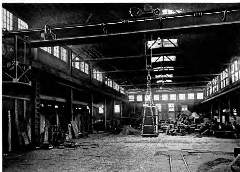
Fig. 29—Method of handling annealing pots with an overhead crane
