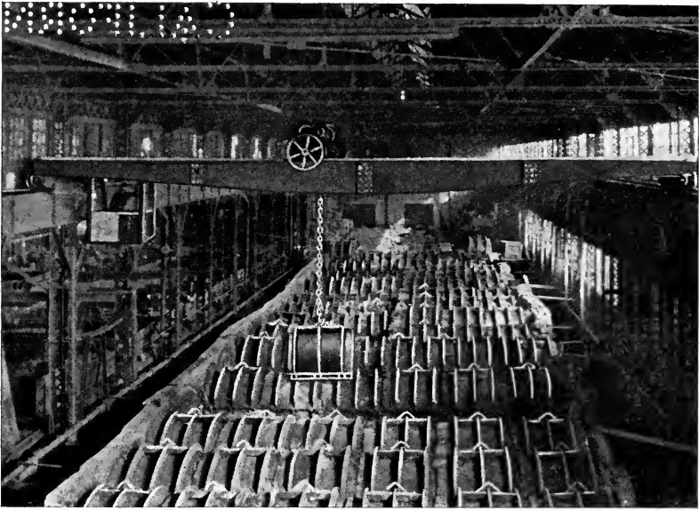
Fig. 26—Annealing furnace located in a concrete pit below the foundry floor level. From the crane is suspended a section of one of the furnace tops
