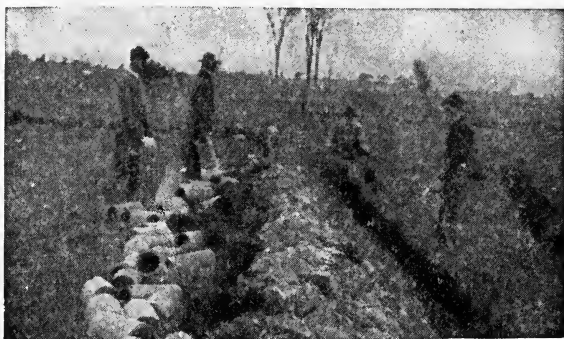
FIG. 38.—Ready to lay the six-inch drain tiles.
