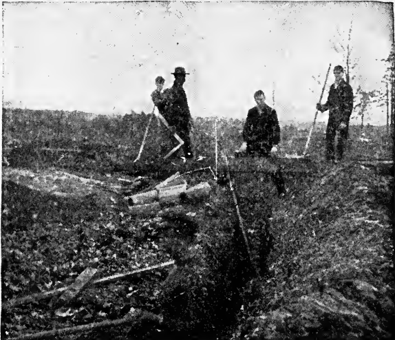
FIG. 40.—Laying drain tiles and testing the depth by measurement from level grade stakes.
