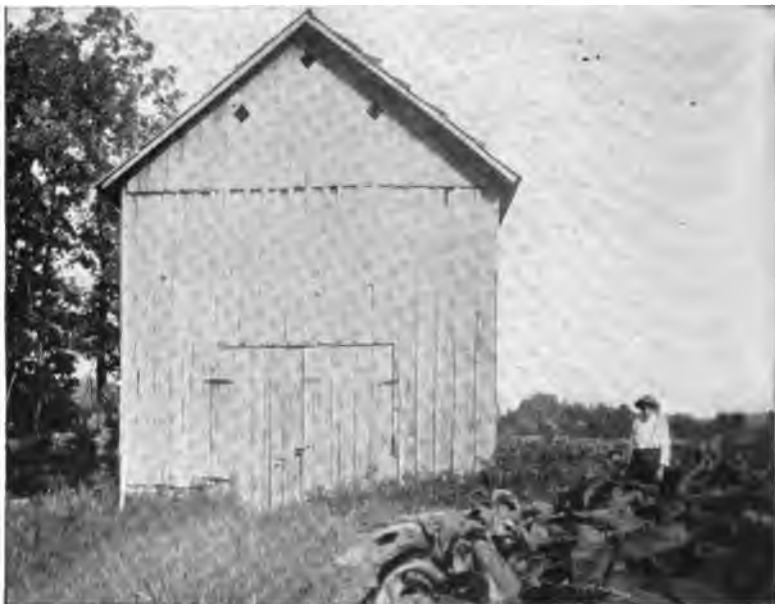
FIG. 259.—Tennessee tobacco barn used in curing dark tobacco, by fire process of removing the moisture. (Productive Farm Crops.)
