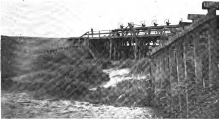
FIG. 87.—A dam of wood and earth erected by private capital to irrigate land to be sold to users. The water "shares" go with the land.
