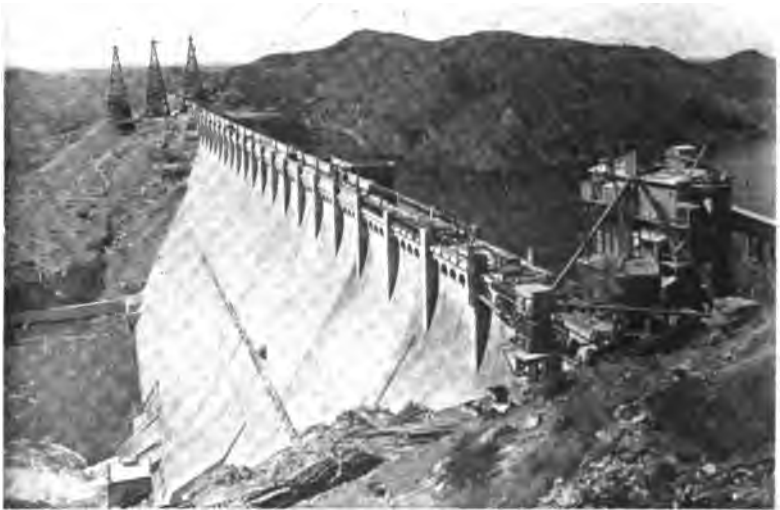
FIG. 88.—Elephant Butte dam, Messila Valley, New Mexico, completed May 13, 1916. It is one of the largest re-enforced concrete dams of the United States Reclamation Service. In these projects the land is sold in small tracts to actual settlers only. (Courtesy Country Gentleman.)
