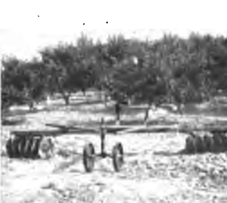
FIG. 218.—The cutaway disk harrow with extension bar and truck. (New Jersey Station.)
