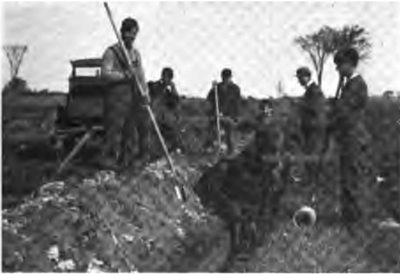
FIG. 85.—Students placing tile in ditch for land drainage.
