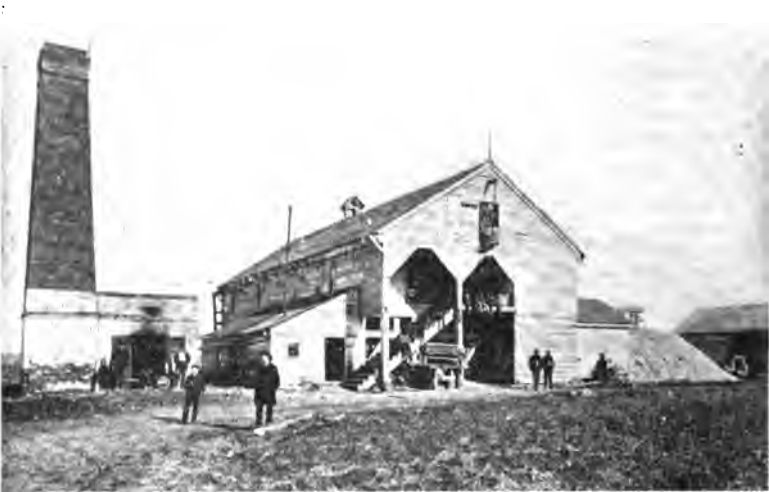
FIG. 194.—A typical cotton-gin house in the rural district of the cotton belt. Note the basket of loose cotton entering at the top. After ginning the fibre is baled. The seeds piled at the rear of the house may be stored in the shed until taken to the oil press. (U. S. D. A.)
