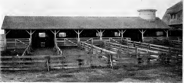
FIG. 237.—Shed, open on one side, University of Illinois; foreground showing fences made of movable panels.
