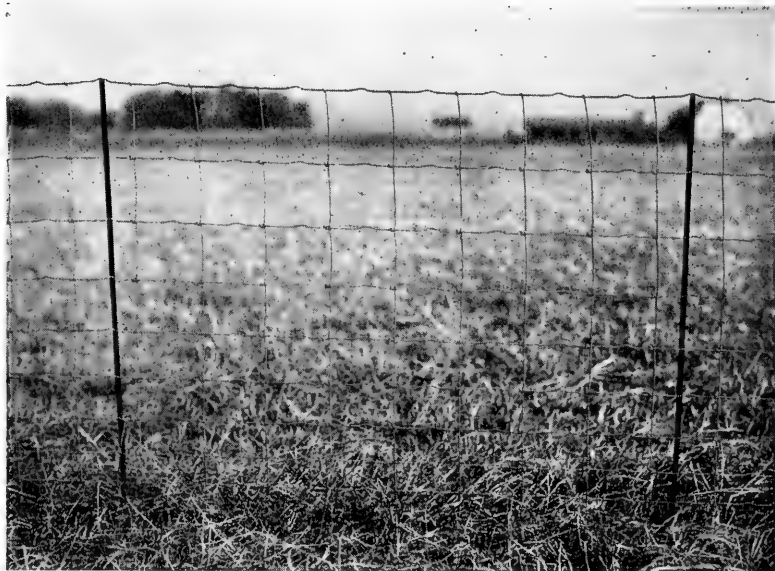
FIG. 251.—Temporary fence supported by iron posts.
