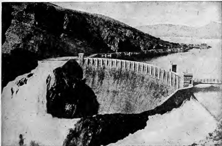
FIG. 64.—Roosevelt Dam, Salt River, Arizona. One of the big dams of the world. Date of construction, 1905-11. Approximate cost, $10,000,000. Used to irrigate 219,000 acres. (U. S. Reclamation Service.)
