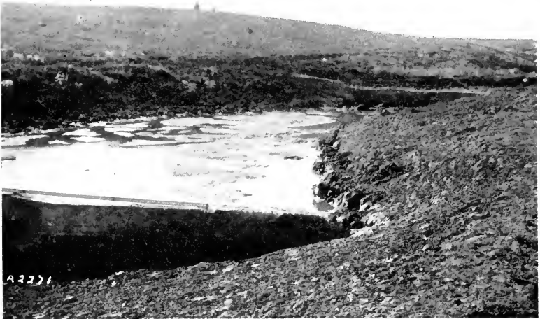
FIG. 193.—Filling a bad gully by means of dams. (Iowa Station.)
