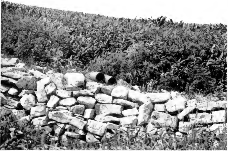
FIG. 192.—A stone dam is effective in filling gullies. (Iowa Station.)
