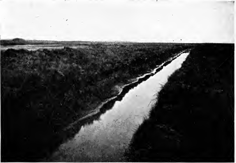
FIG. 50.—A good outlet ditch. This was dug with a floating dredge. It is 20 feet wide at the top and 7 feet deep. (Wisconsin Station.)
