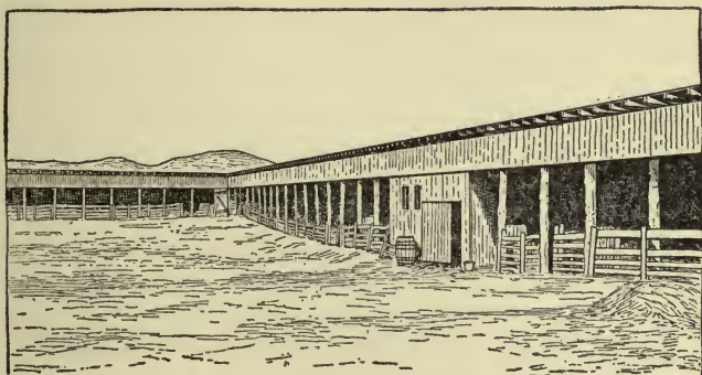
AN IDAHO LAMBING SHED
