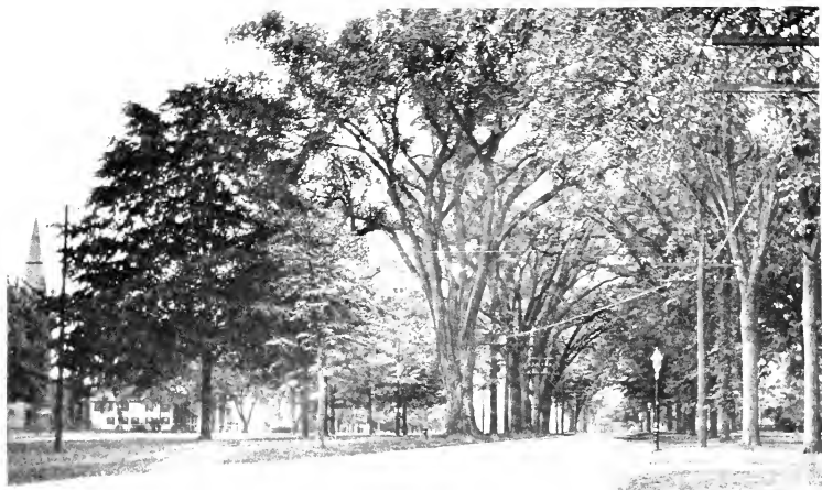
LONGMEADOW BOULEVARD, the beautiful suburb, being rapidly built up by Springfield people.
