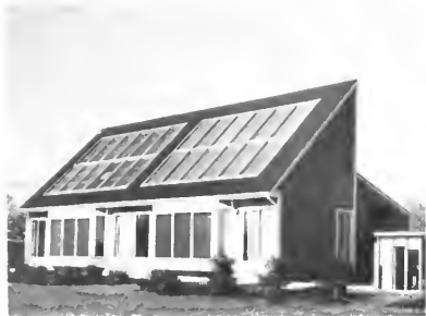
An experimental solar house. Glass panels trap heat through the greenhouse effect. Solar cells beneath the panels convert light to electricity, which can then be stored in batteries. Heat from the cells is transferred to a coolant and stored for later use.
