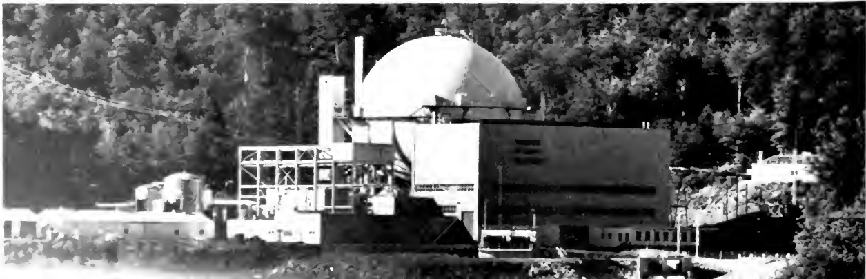
The Yankee Atomic Electric nuclear power station in Rowe, Massachusetts, which has been producing electricity with a capacity of 175,000 kW since 1961.
