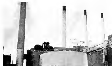
A typical fossil-fuel power plant that produces electricity by burning coal.
