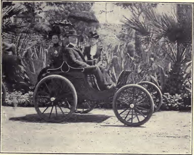
FIG. 68.—Duryea Four-wheeled Trap. This carriage, like all others made by the Duryeas, has no underframe; the strongly built body serving as a frame to which the axles and springs are hung.
