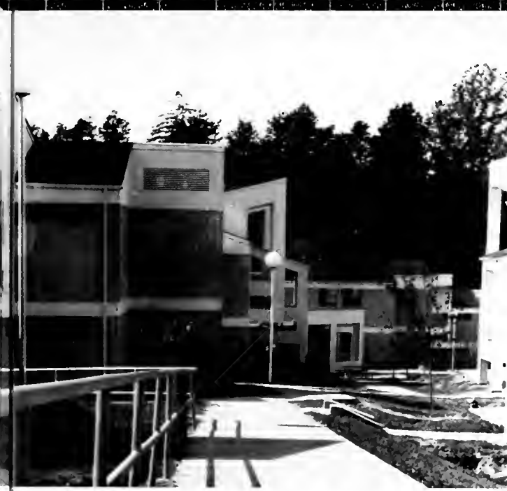
Top Left. UNCC's newest on campus housing: Hawthorne Hall. Lower: Roommates, ya' know 'em, ya' love 'em, you can't live without 'em, unless you pay one and a half housing. Top Right: The luxurious Phase III apartment complex. Center Right: A familiar sight to Phase II students. Lower Right: Socializing outside Phase IV A.
