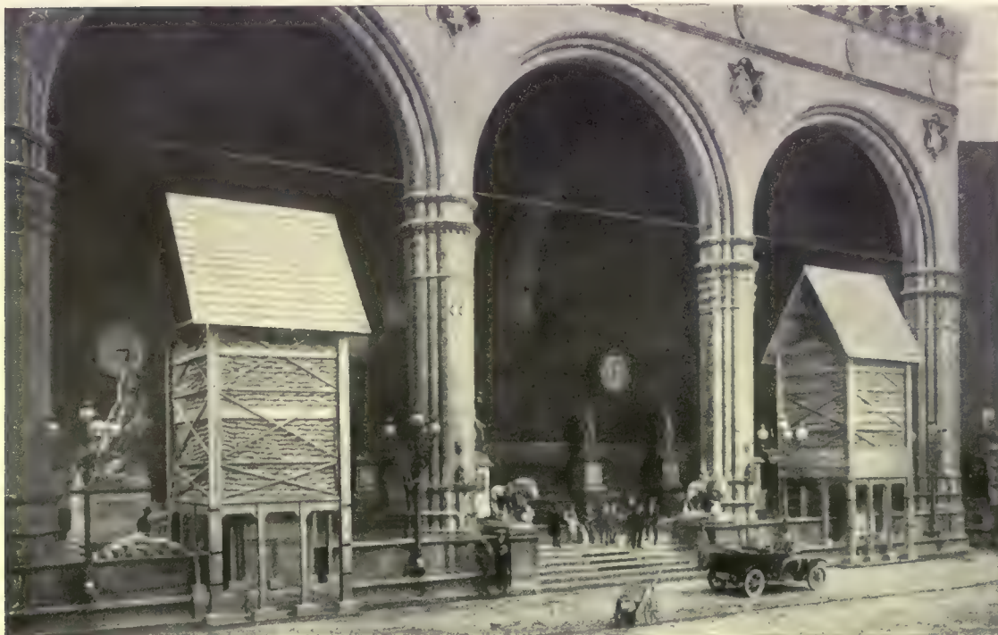
Florence. The Loggia dei Lanzi with the protection for the sculptures by Benvenuto Cellini and Giovanni da Bologna
