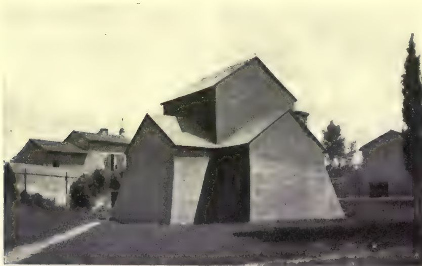
Ravenna. Protection of the Mausoleum of Galla Placidia
