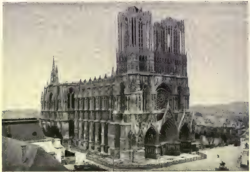
Reims. The Cathedral after the fire. This shows that even after the fire in the roof the whole architectonic form was intact and that the Cathedral was in no way a "heap of ruins"
