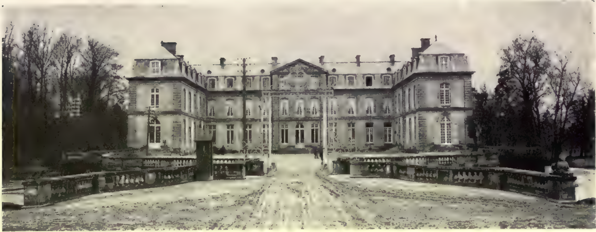
Castle of Pinon before its destruction
