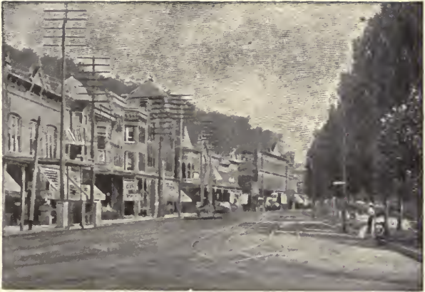
CENTRAL AVENUE, LOOKING NORTH.
