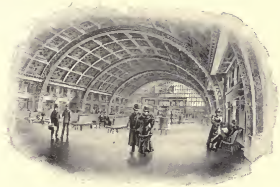
INTERIOR CHICAGO STATION.
