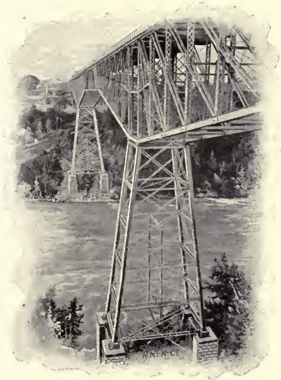
THE CANTALIVER BRIDGE MICHIGAN CENTRAL RAILROAD
