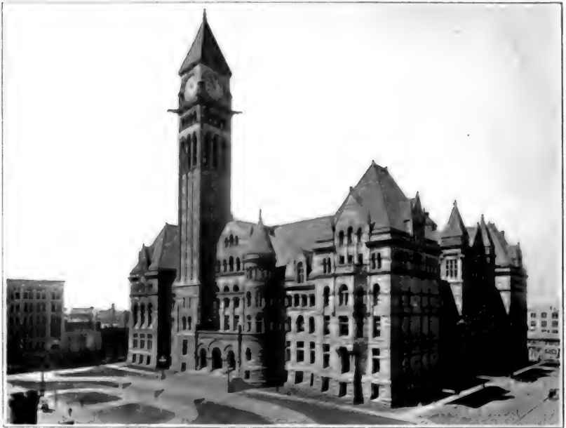
Municipal Buildings, Toronto.
