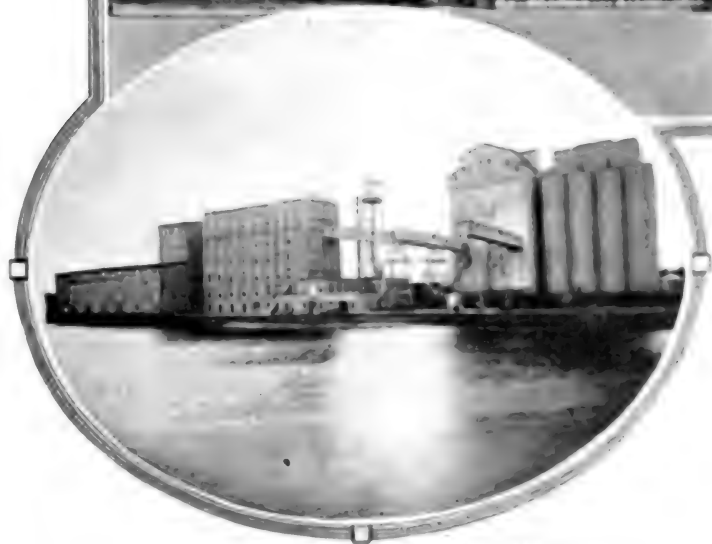
G. I. P. Elevator - Flour Mill Fort William
