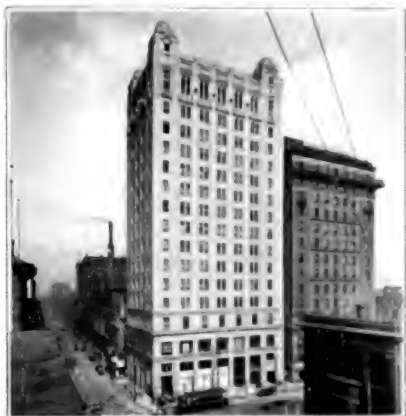
C.P.R. Offices, Toronto, 237 ft. high, the highest office building in the Empire.
