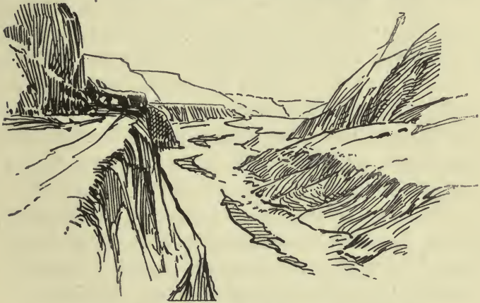
CONSTRUCTION DAYS IN CULEBRA-GAILARD CUT
