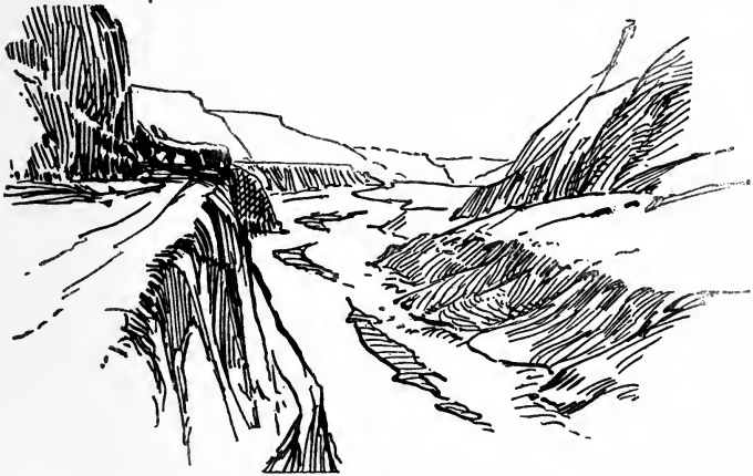
CONSTRUCTION DAYS IN CULEBRA-GAILLARD CUT
