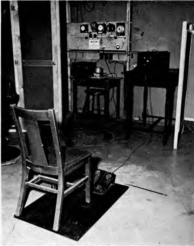
Fig. 5. A Serial Reaction Apparatus. The subject sits on the chair with his foot on the pedal and reacts to one of three lights, red, green, or orange. If red appears he is to shift his foot quickly to the other pedal. The time is measured. If green appears and the subject shifts his foot, an error is recorded. The orange light is the warning signal. (After Stalder.)
