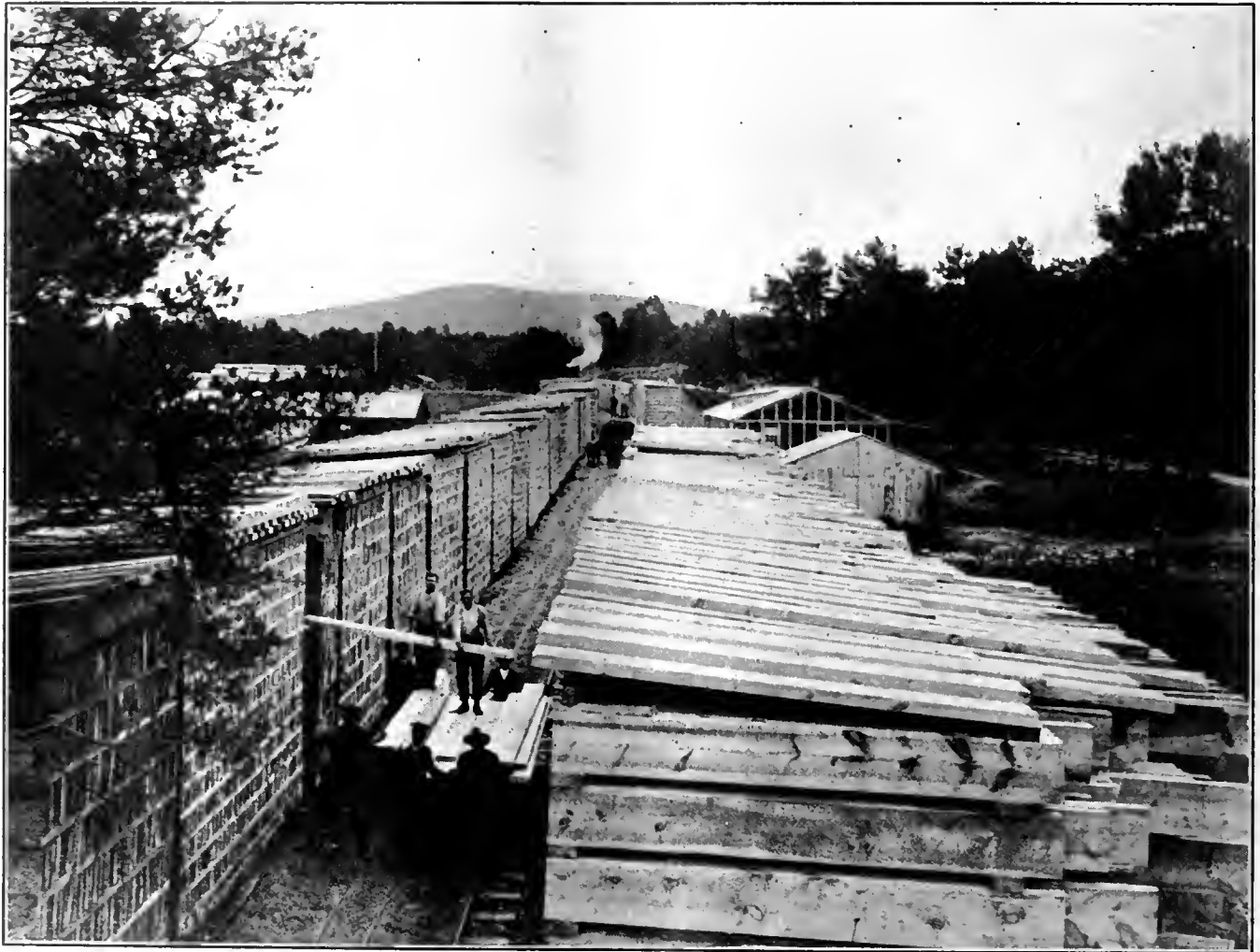
TIMBER STACKS AT A CANADIAN CAMP
