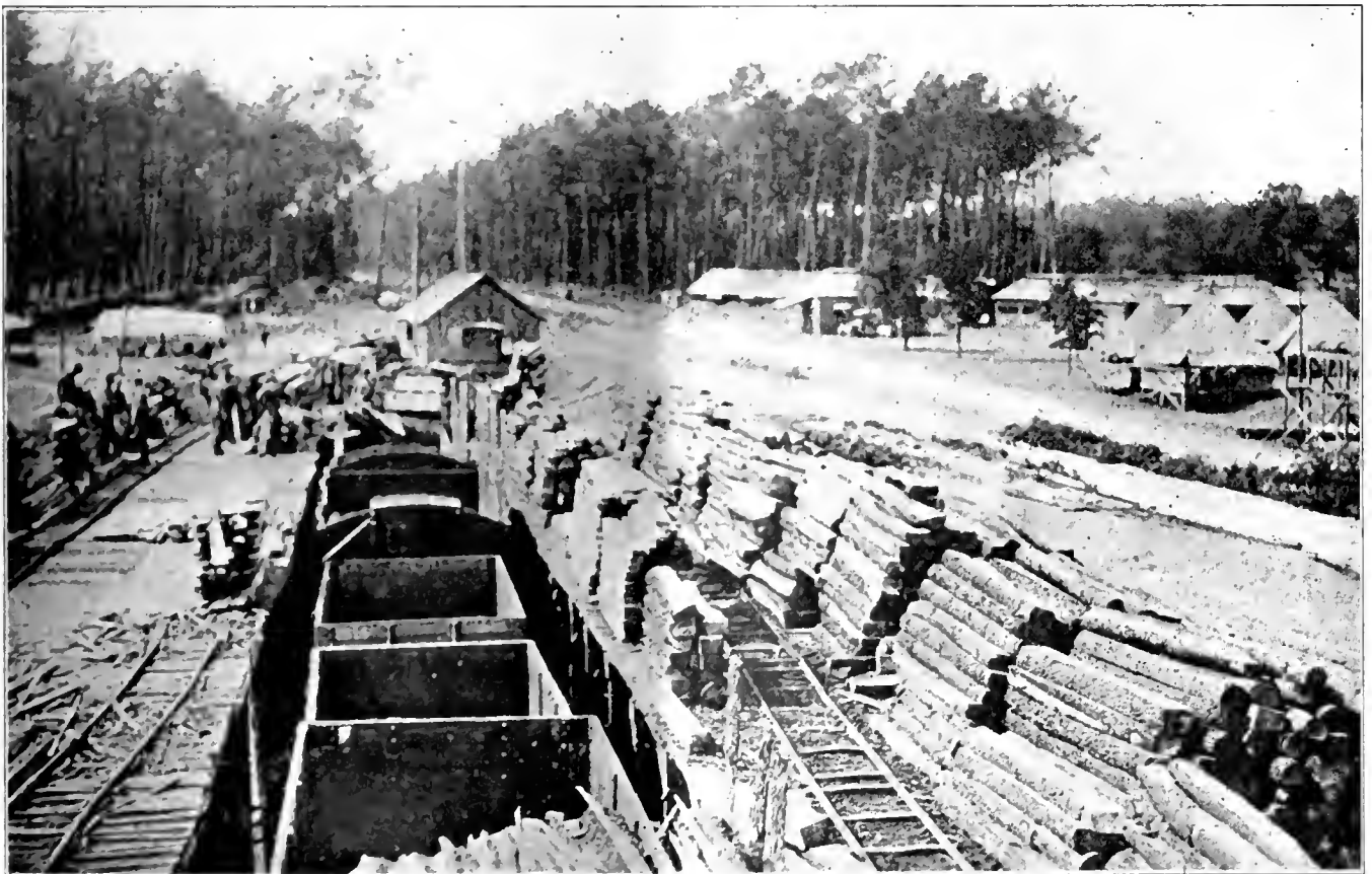
SCENE IN A MARITIME PINE FOREST, SOUTHWESTERN FRANCE. BROAD GAUGE SPUR PARALLELED BY LOADING DOCKS ON WHICH ARE NARROW GAUGE TRACKS TO TRANSPORT TIES AND OTHER PRODUCTS FROM THE MILL TO THE FRENCH RAILWAY CARS IN THE CENTER
