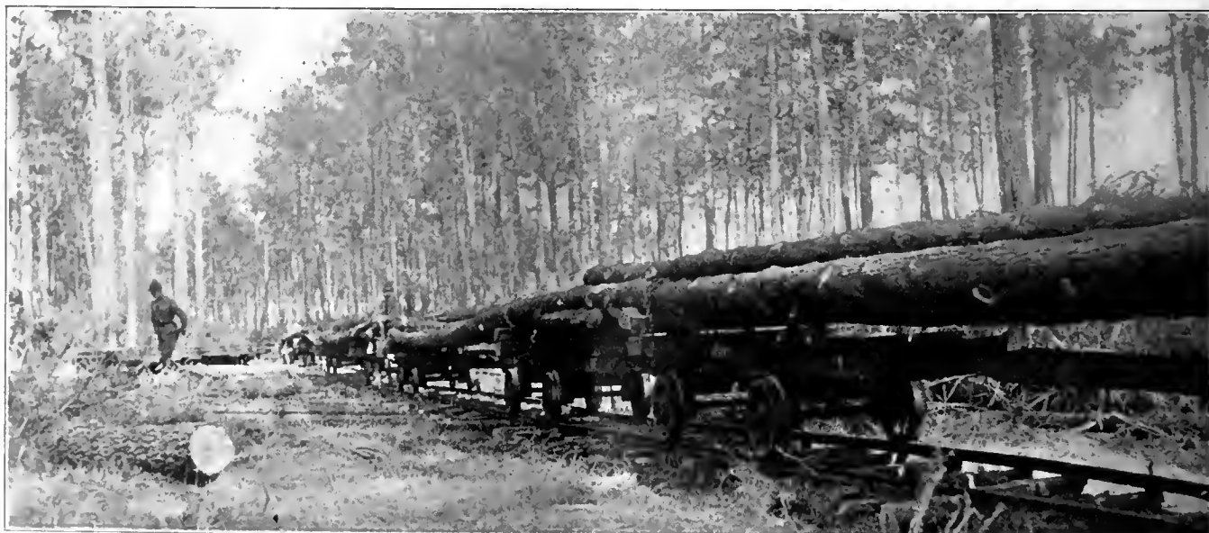
LONG MARITIME PILING LOADED ON AMERICAN NARROW GAUGE CARS READY FOR TRANSPORTATION FROM THE FOREST TO THE MAIN LINE RAILWAY SHIPPING POINT NEAR PONTENX, LANDES, FRANCE
