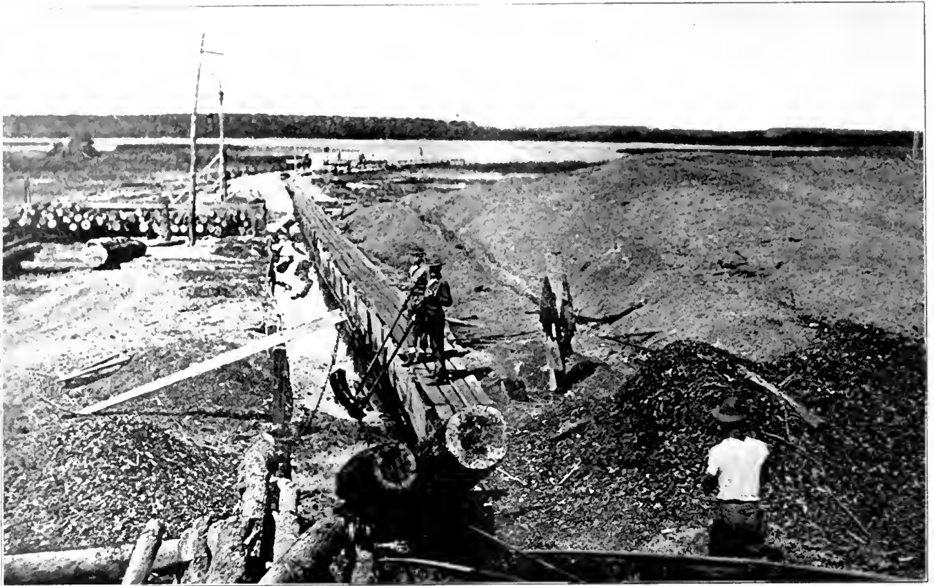
VIEW OF AUREILHAN LAKE, FRANCE, FROM AMERICAN 20-M SAWMILL. LOGS WERE TOWED ACROSS THE LAKE FROM THE MOUTH OF THE COURANT RIVER, BROUGHT TO THE BOOMS AT THE EDGE OF THE LAKE, THEN POLED ALONG THE CANAL TO THE POINT IN THE FOREGROUND WHERE THEY WERE LOADED UPON A SMALL CAR WHICH WAS PULLED BY CABLE UP THE INCLINE INTO THE SAWMILL. THE LARGE HEAP OF SAWDUST AT THE RIGHT WAS PRODUCED BY THE MILL AS THE RESULT OF SEVERAL MONTHS' OPERATION
