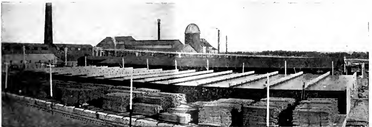
Showing 14 Moore Moist Air Kilns (they are operating a total of 34 Moore Kilns) at plant of Atlantic Coast Lumber Corp., Georgetown, S. C., on the Atlantic Coast. This is the largest board mill in the world, having a daily capacity of three-quarters of a million feet in boards.
