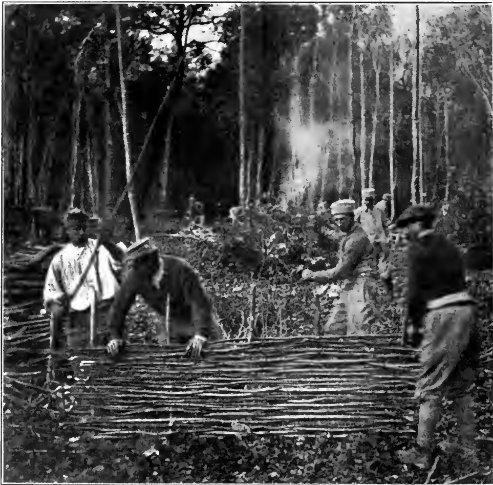
WEAVING SUPPORTS FOR SIDES OF TRENCHES
