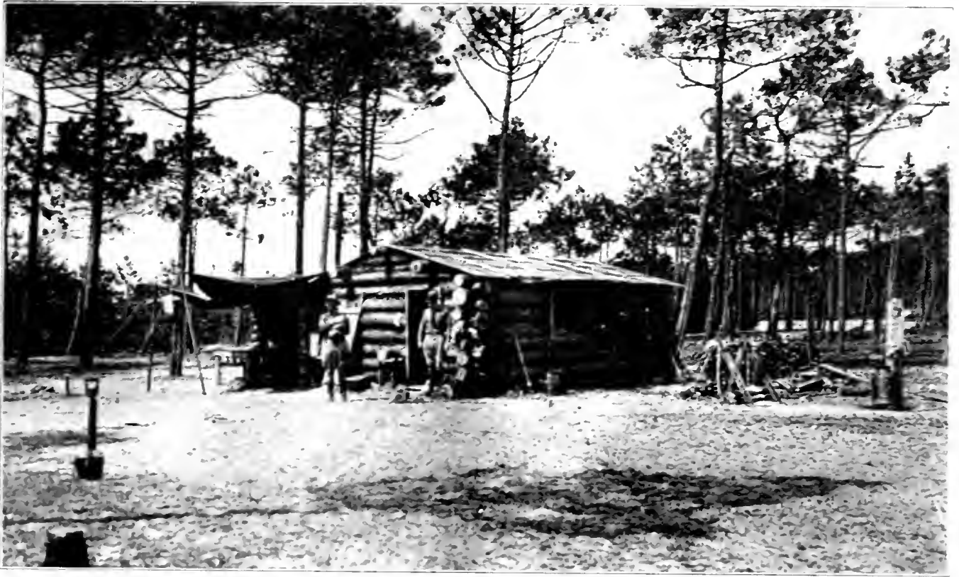
A LOG CABIN BUILT NEAR PONTENY, LANDES, FRANCE, BY A SQUAD OF AMERICAN RIVER DRIVERS IN THE 29th REGIMENT. THE FRENCH NEVER USE WOOD SO LAVISHLY IN BUILDING
