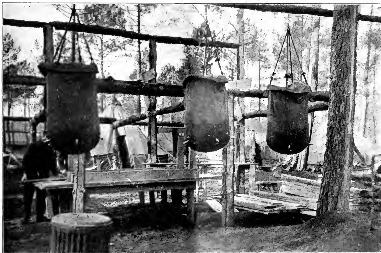
LISTER BAGS ("CARRIE NATION COWS") CONTAINING CHLORINATED WATER FOR DRINKING PURPOSES. BELLEVUE CAMP, PONTENX, LANDES, FRANCE
