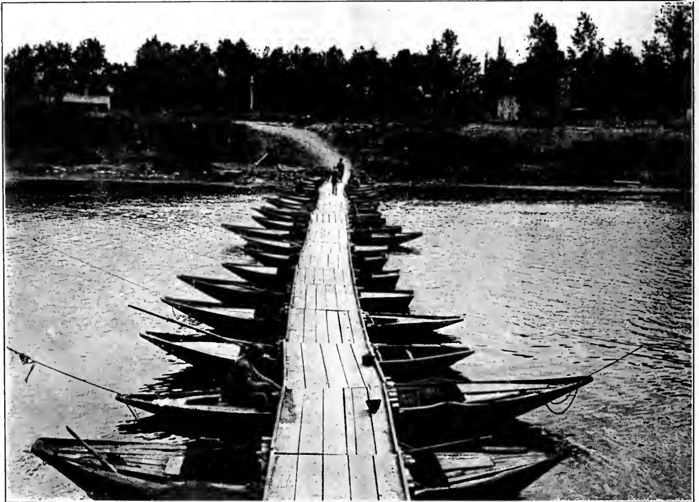
A PONTOON BRIDGE ACROSS THE MARNE
