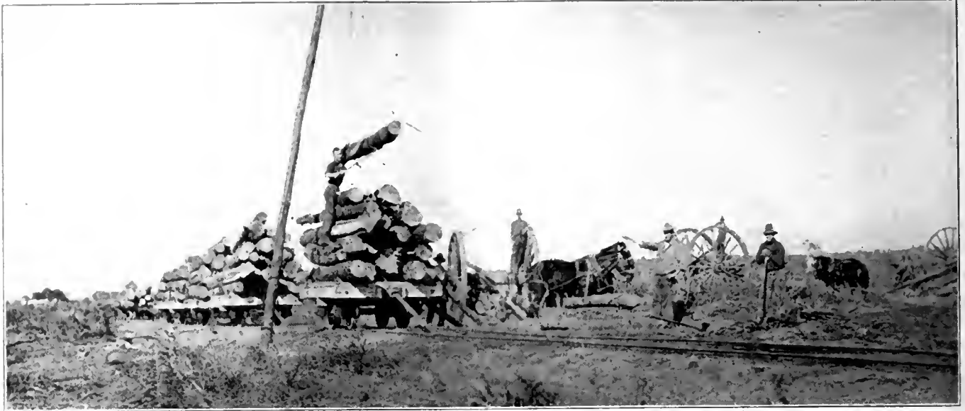
LOADING MARITIME PINE LOGS ON NARROW GAUGE RAILWAY CARS FOR TRANSPORTATION TO AMERICAN 20-M MILLS IN SOUTHWESTERN FRANCE. THE PINE FOREST IS HERE CUT CLEAN. BIG WHEELS USED TO SKID LOGS TO THE RAILWAY SHOWN AT THE RIGHT
