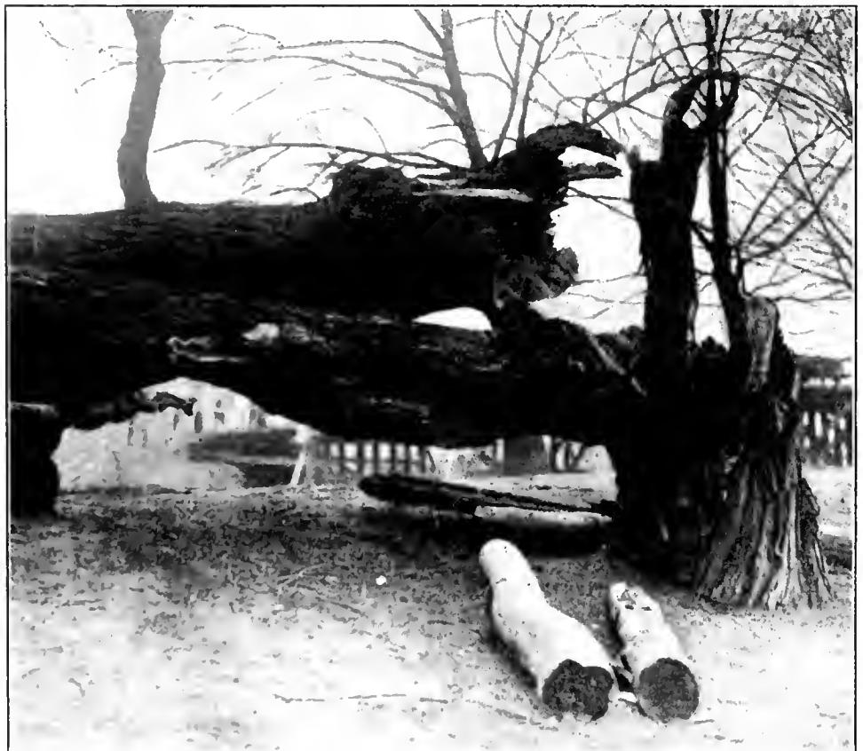
Underwood and Underwood DAMAGED CAUSED BY ONE SHELL
