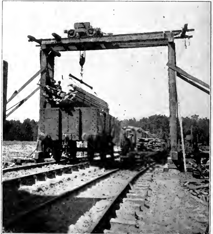
THESE LOADING CRANES WERE USED FOR TRANSFERRING THE LUMBER FROM NARROW GAUGE TO BROAD GAUGE CARS IN MANY OF THE SHIPPING YARDS OF THE 20th REGIMENT
