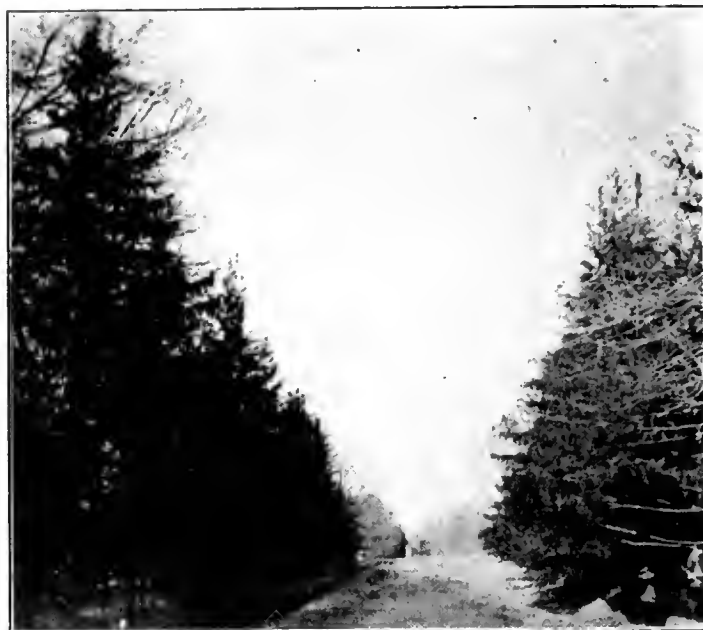
LOOKING UP THE AQUEDUCT NEAR THE GOULD ESTATE
