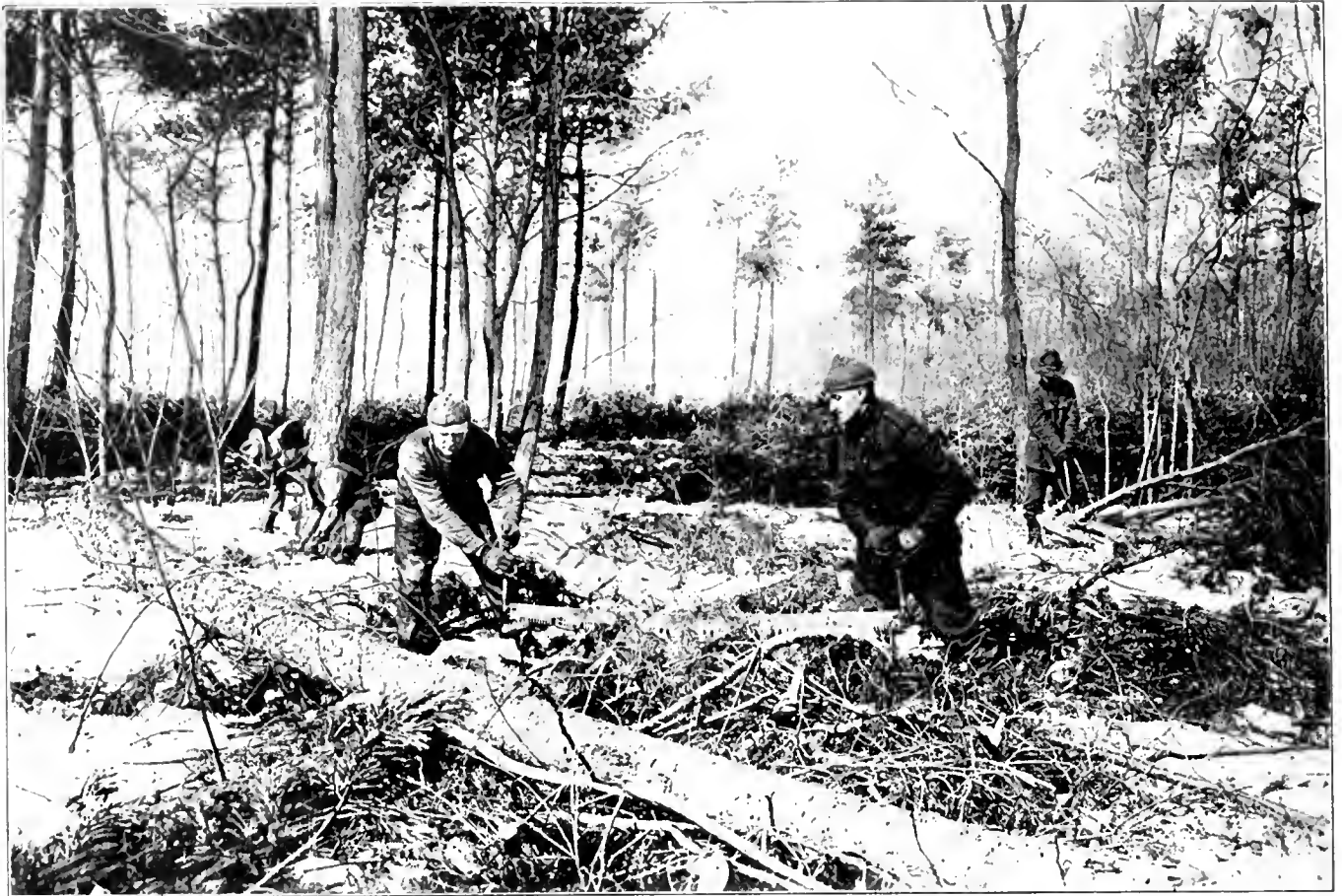
30th ENGINEERS SAWING FELLEED TREES INTO LOGS IN A PINE FOREST, SOUTHERN FRANCE
