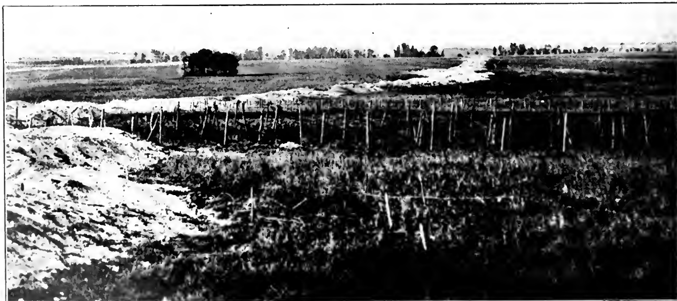
SMALL POSTS USED FOR WIRE ENTANGLEMENTS
