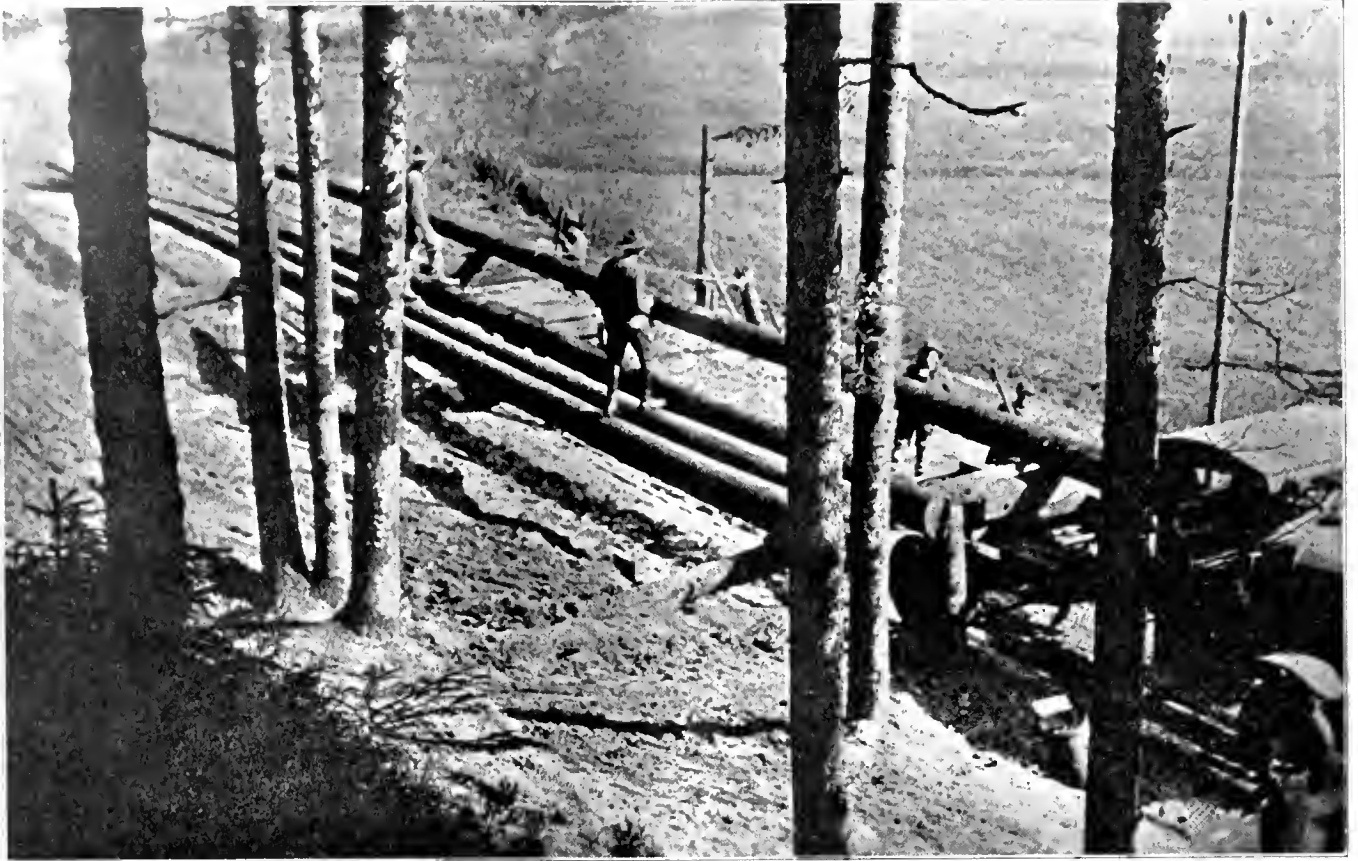
MEMBERS OF THE 20th ENGINEERS LOADING PILING ON TRUCKS AT LANDING No. 2 IN FRANCE. THESE PILING ARE APPROXIMATELY SEVENTY FEET LONG
