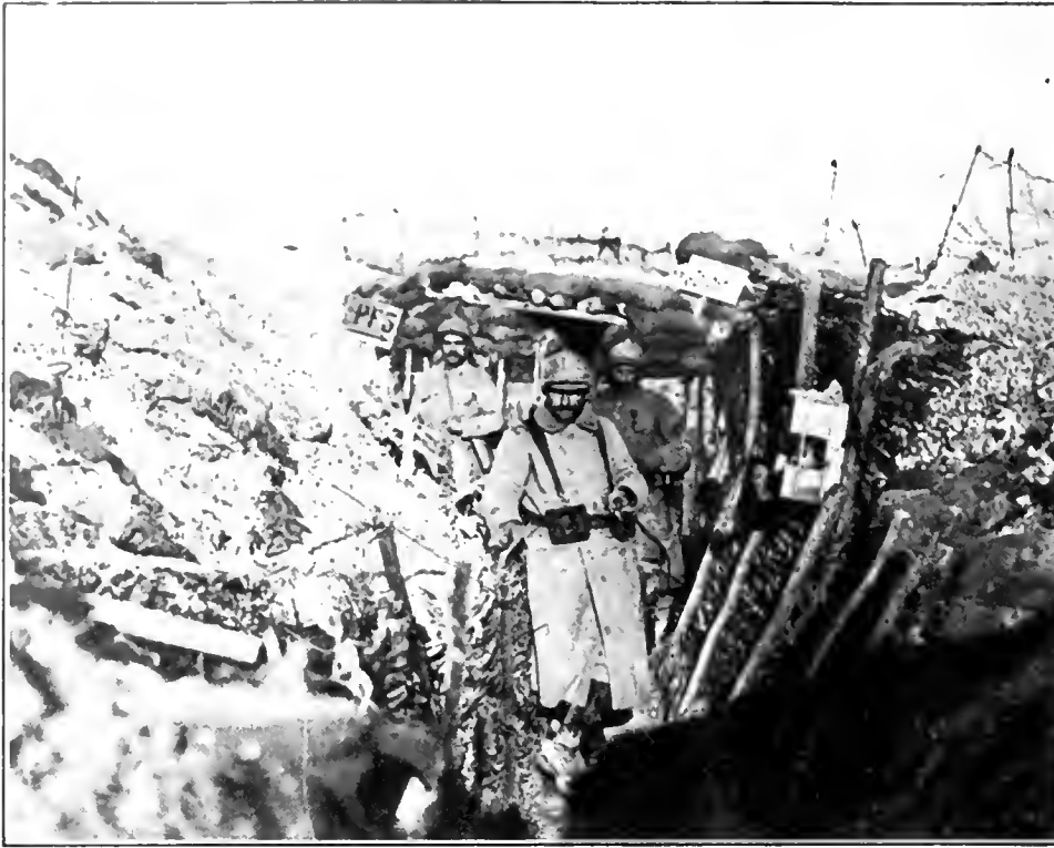
LUMBER USED IN TRENCH CONSTRUCTION
