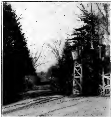
THE AQUEDUCT, CROSSING SUNNYSIDE LANE
