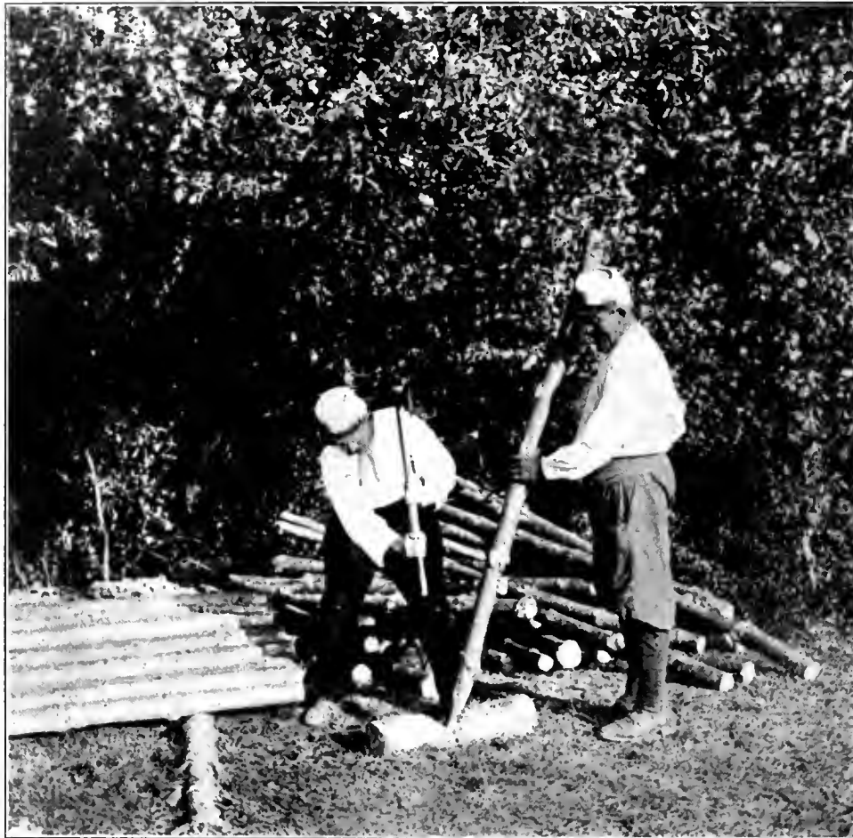
CUTTING AND SHARPENING BARBED WIRE STAKES
