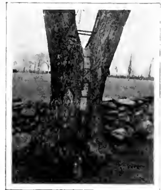
Note that the concrete filling is laid in sections, thus forming "rocking joints" which allow for swaying and prevent cracking. Rigid steel rods bind the branches at the crotch firmly together
