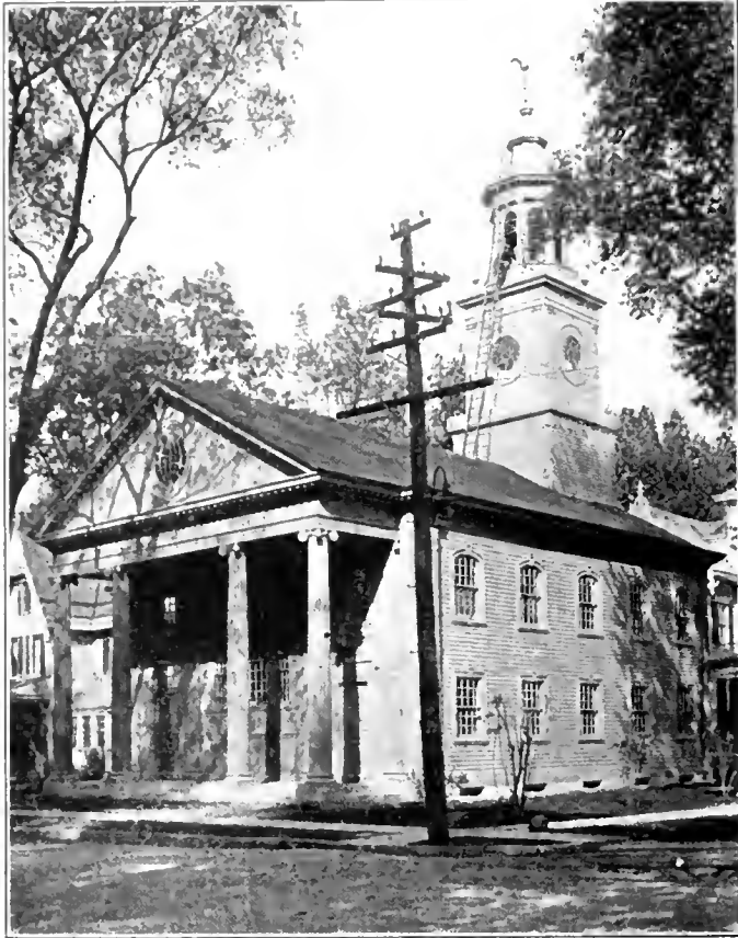
THE EXTERIOR OF THE BUILDING
