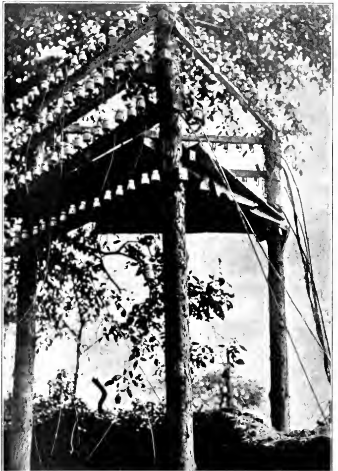
THE LUMBERJACKS AND FORESTERS HELPED TO BUILD TELEPHONE SYSTEM PLATFORMS IN FRANCE WHICH WERE LIKE FIRE LOOKOUT STATIONS IN OUR OWN FORESTS.
