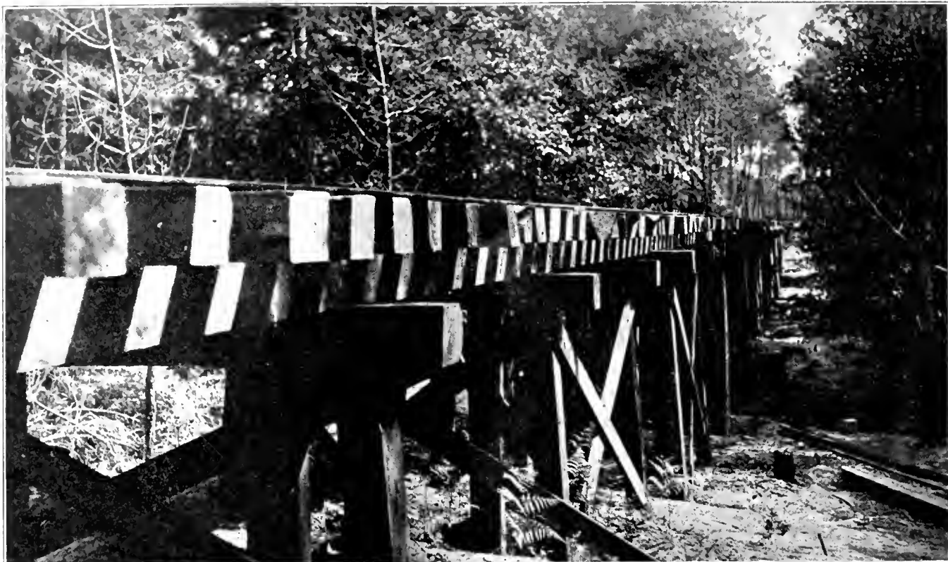
PORTIONS OF TRESTLE BUILT BY THE 20th ENGINEERS IN THE MARITIME PINE FOREST IN THE LANDES, IN SOUTHWESTERN FRANCE TO TRANSPORT FOREST PRODUCTS FROM THE WOODS TO THE MAIN LINE
