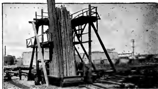
Consumer's Open Tank process (hot and cooling treatment) cedar pole creosoting plant.
