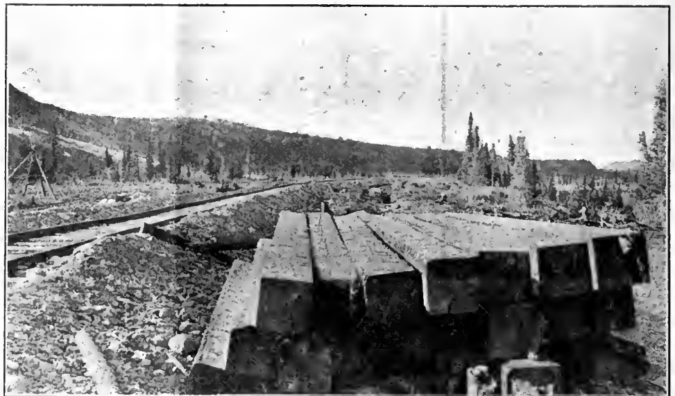
WHITE SPRUCE BRIDGE TIMBERS CUT ALONG RIGHT OF WAY, NEAR HEALY, AT THE END OF STEEL ON THE GOVERNMENT ROAD
