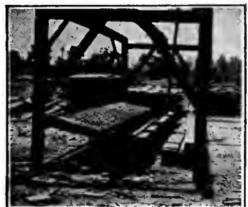
Single unit tank for creosoting coal mine shaft timber. Built of tongue and groove lumber, double wall, caulked, etc. Metal lining is preferable to guard against leakage.
