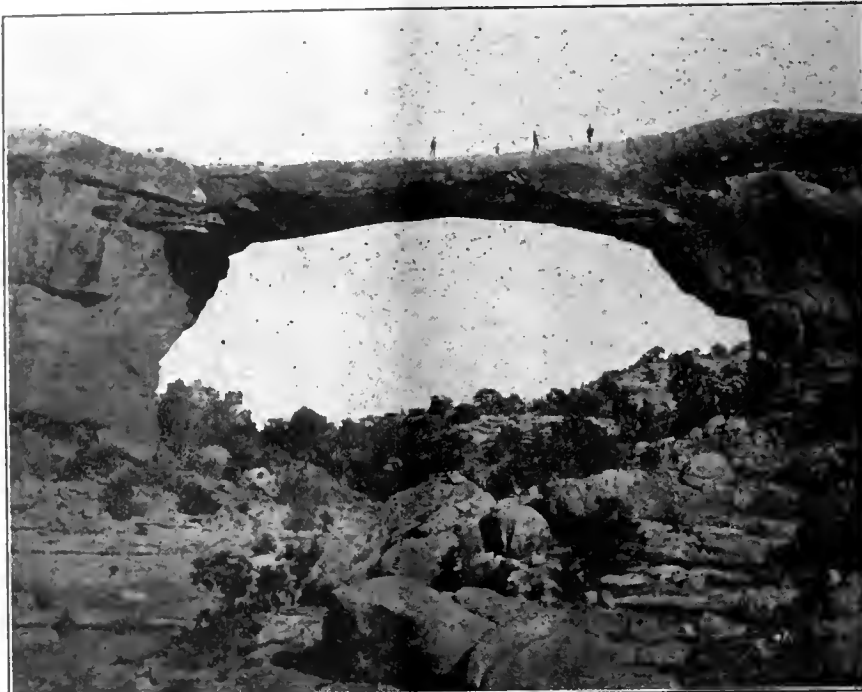
THE EDWIN NATURAL BRIDGE
