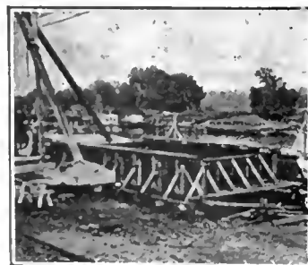
Single unit plant for hot and cooling treatment. Wood tank, lined with sheet metal, equipped with steam coils. Capacity: 10,000 ft. B. M., per 24 hour day.
