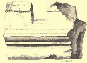
Fig. 5. Part of Parapet.
