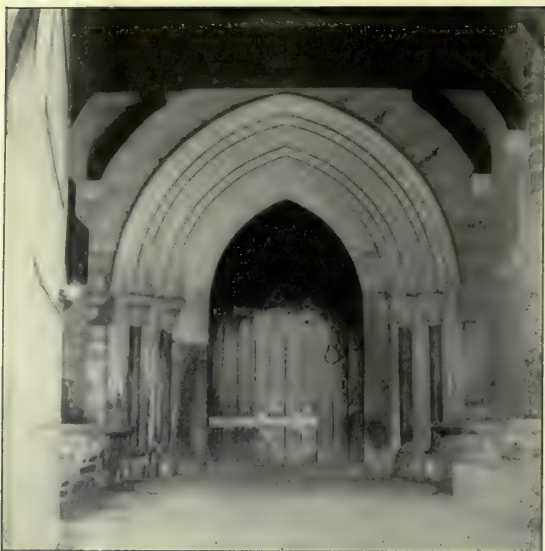
Inner Door of North Porch.
