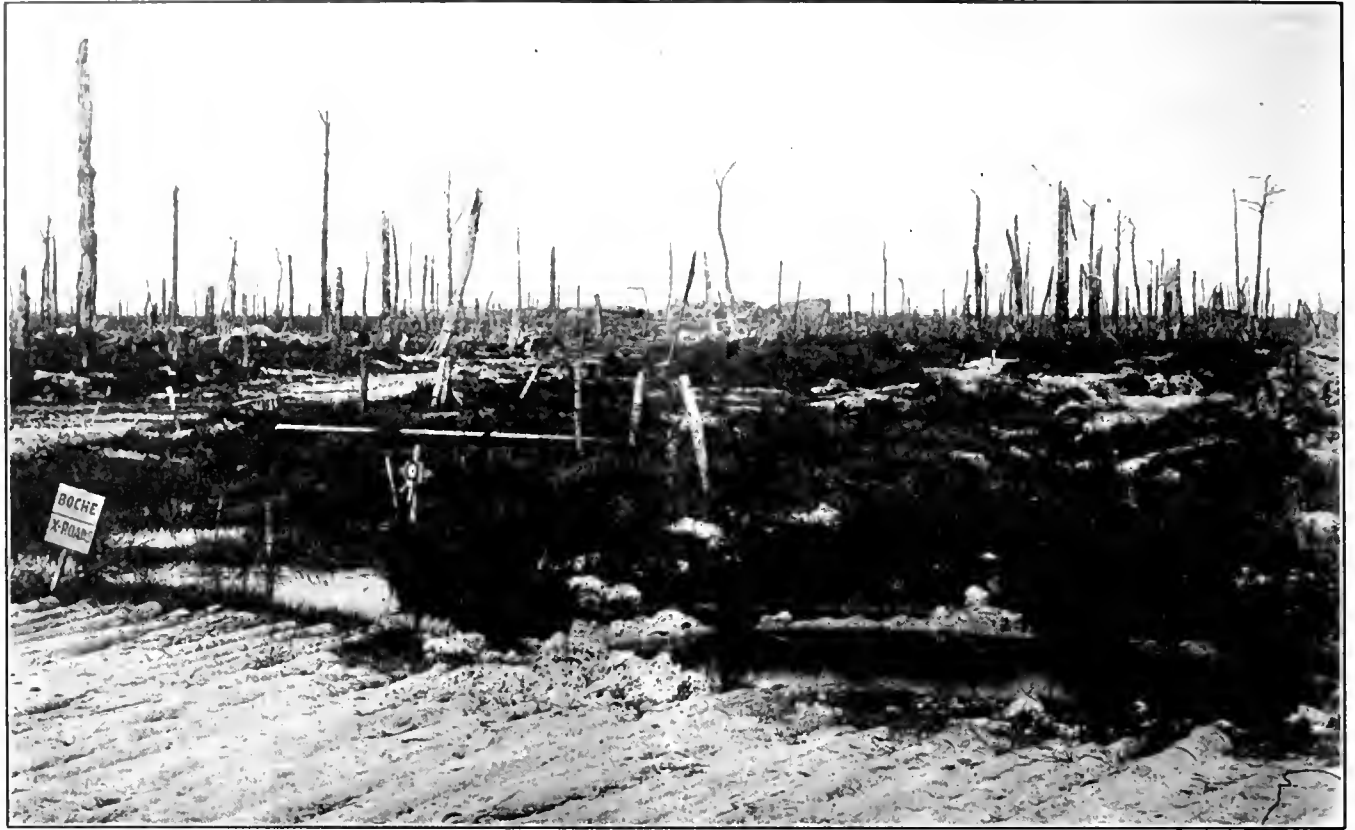
THIS SCENE NEAR BOESINGHE, BELGIUM, INDICATES HOW THE GERMANS USED VAST QUANTITIES OF BELGIAN TIMBER IN BUILDING ROADS ON LOW GROUND. THE TREES STILL STANDING ARE DEAD, SHATTERED BY SHELL AND GUN FIRE.
