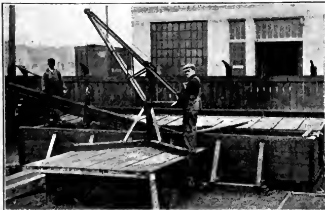
The Open-Tank Process: Simple wooden tank (lined with sheet iron) equipped with steam-coils and small derrick. Upon expiration of the hot treatment, both oil and timber are permitted to cool instead of being transferred to a cold tank. Fence surrounding this plant has been creosoted.
