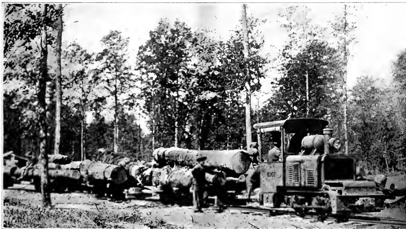
A TRAINLOAD OF LARGE HARDWOOD LOGS CUT FROM ONE OF THE ROTHSCHILD ESTATES BY THE 20th ENGINEERS
