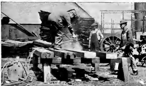
Applying surface treatment by spraying Carbosota on contact surfaces.
