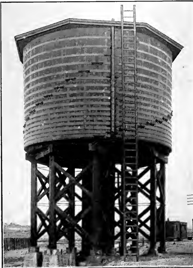
Knowles Type Creosoted Water Tank erected at Mattoon, Ill., by the Illinois Central R.R. (Creosoted by Empty-Cell-Rueping Process 5 lbs. A.R.E.A. No. 1 Coal-Tar Creosote Oil per cubic foot.)
