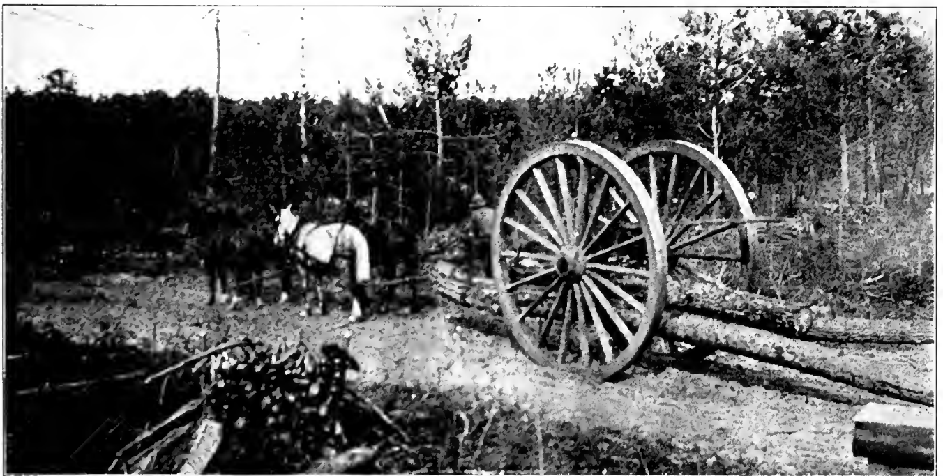
20th REGIMENT MEN TRANSPORTING LOGS, BY MEANS OF "BIG WHEELS," TO THE BANK OF THE COURANT RIVER, AUREILHAN OPERATION, NEAR PONTENX, LANDES, FRANCE
