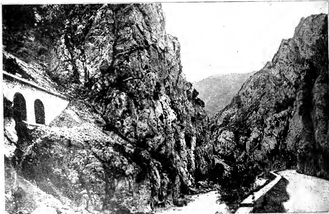
ENTRANCE OF THE RIVER AUDE NEAR QUILLAN, EASTERN PYRENEES, INTO THE GORGE WHICH IT HAS CARVED FOR ITSELF EN ROUTE TO THE SEA (PAGE 1193)
