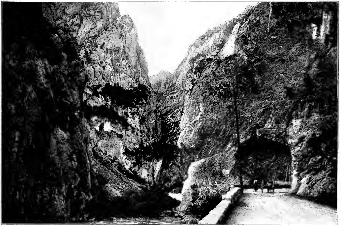
SO NARROW IS THE GORGE THROUGH WHICH FLOWS THE RIVER AUDE, NEAR QUILLAN, IN THE EASTERN PYRENEES, THAT THE ROAD HAD TO BE TUNNELLED THROUGH THE ROCK
