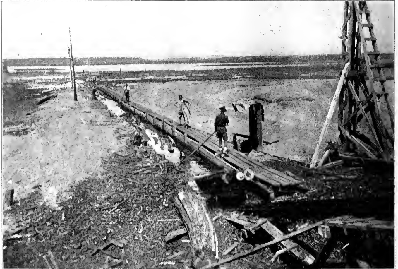
CANAL AND CAR BRINGING LOGS UP TO THE HOIST INTO THE AUREILHAN MILL OF THE 20th ENGINEERS NEAR PONTENX, LANDES, FRANCE
