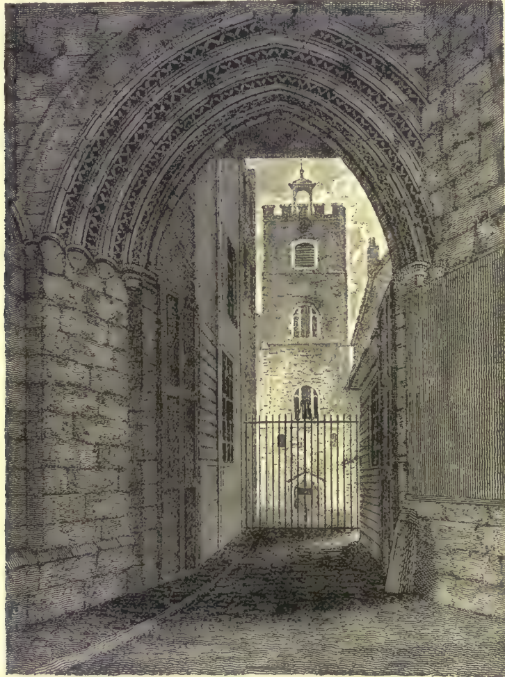
THE GATE OF ST. BARTHOLOMEW'S PRIORY
