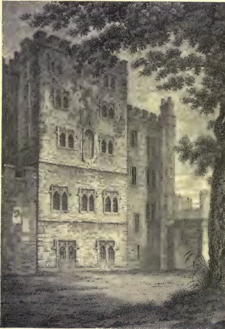
THE LOLLARD'S TOWER, LAMBETH PALACE
