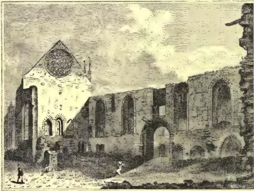
NORTH-WEST VIEW OF THE RUINS OF THE BISHOP OF WINCHESTER'S PALACE, SOUTHWARK
