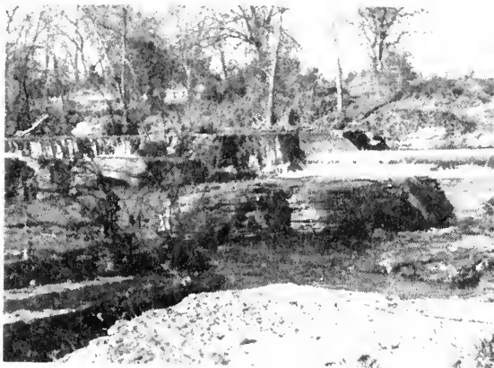
Water flowing through a central gate to the right was channeled into the canal to the mill house. In the foreground was once the dirt creek bank.
