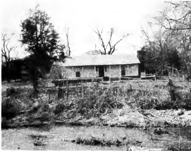
Old house in Big Springs
