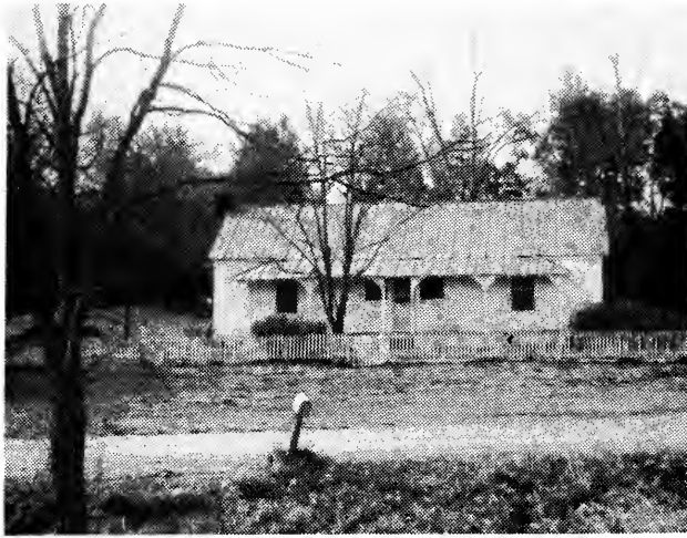
Old house pegged together
