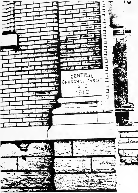
Original cornerstone in the foundation
