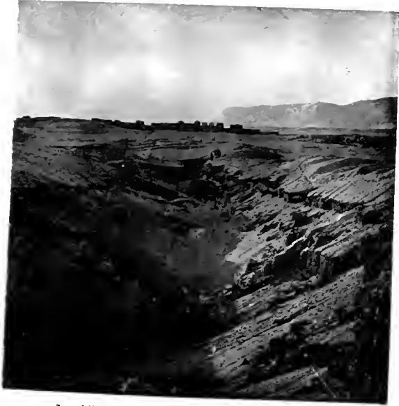
1. VIEW LOOKING SOUTH, SHOWING DIRECTION OF TRENCH.
