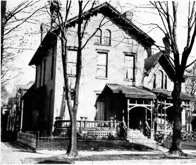
FLAG-DANFORTH HOUSE, NO. 55 ALLEN STREET. TORN DOWN, 1921.
