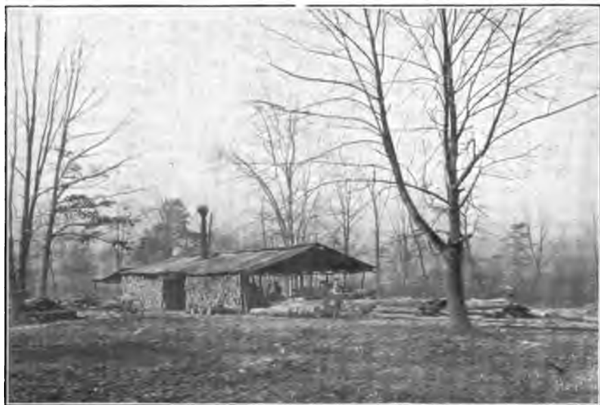
Fig. 63. General view of combination portable saw and shingle mill. A type of mill which will effect closer utilization of blighted chestnut than the saw mill alone.
