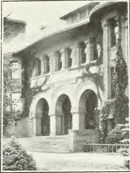
“OLD PALMER’S MASSIVE WALLS”
