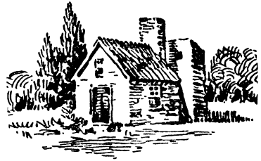
FIG. 4. TOWN SCHOOL AT DEDHAM, MASSACHUSETTS, BUILT IN 1648
