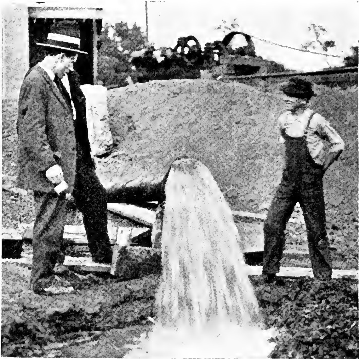
TESTING A DRIVE WELL
