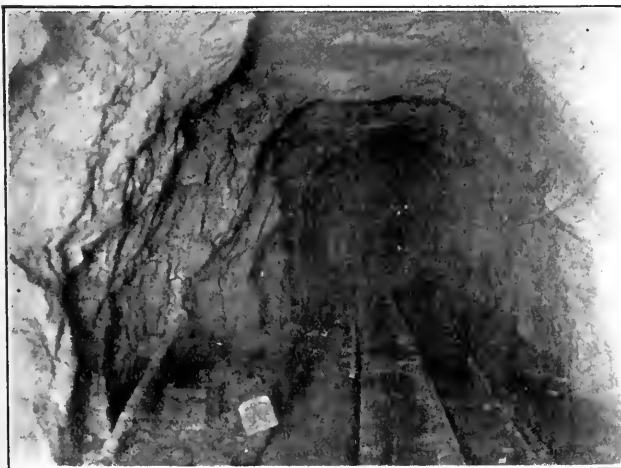
ROCK TUNNEL, RIVER DES PERES SEWER
