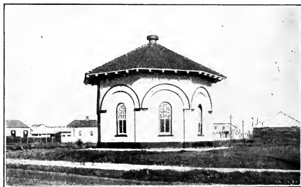
SUB-STATION NO. 14, SEWAGE PUMPING
