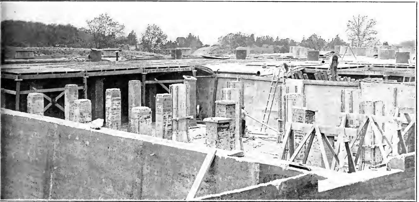
PEEKSKILL FILTERS PARTLY ROOFED OVER
