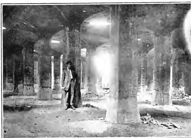
INTERIOR OF FILTER, MASONRY COMPLETED
