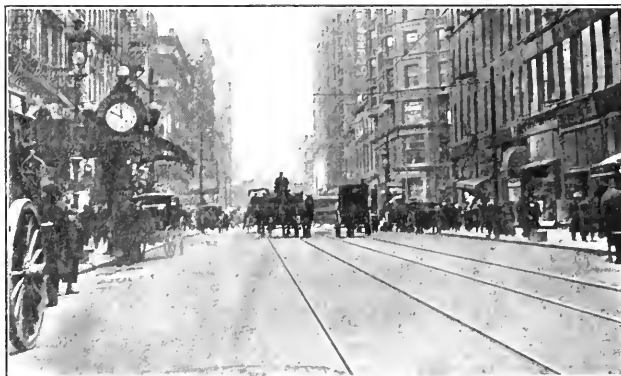
MADISON STREET, CHICAGO. WOOD BLOCK PAVING.
