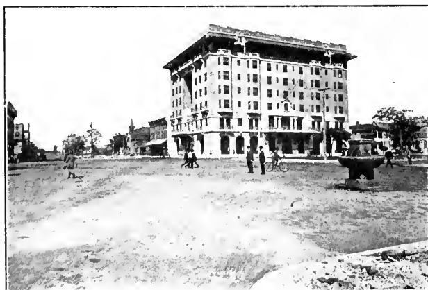
INTERSECTION WITHOUT EXPANSION JOINTS
