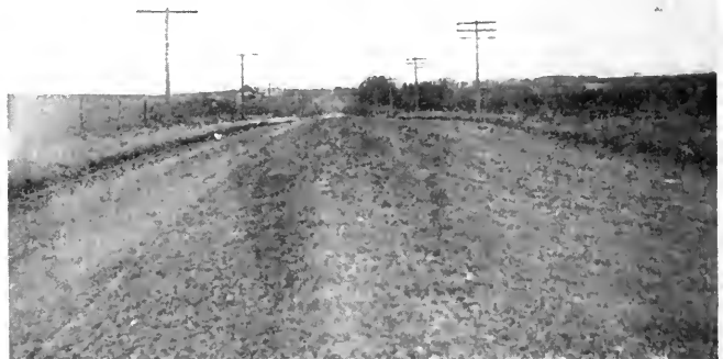
STRETCH OF FINISHED ROAD
