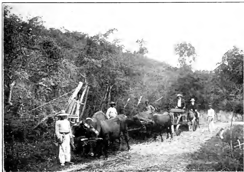
BUILDING ROAD IN WEST INDIES WITH OHIO REVERSIBLE ROAD GRADER.
