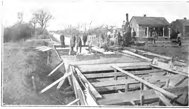
FORMS FOR CONDUIT WALLS IN PLACE Outside forms braced against bank.
