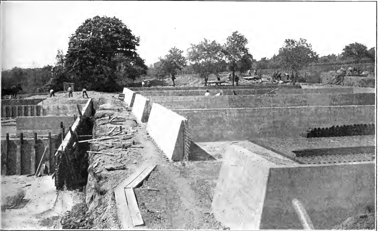
FIG. 1. PRIMARY AND SECONDARY CONTACT BEDS UNDER CONSTRUCTION
