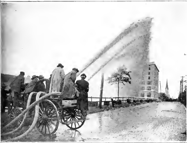
Courtesy the Florida Times-Union. TESTING HIGH-PRESSURE SYSTEM
