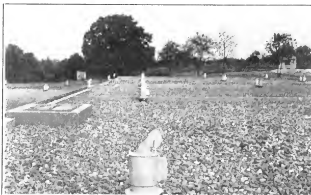
FIG. 8. PRIMARY CONTACT BEDS COMPLETED
