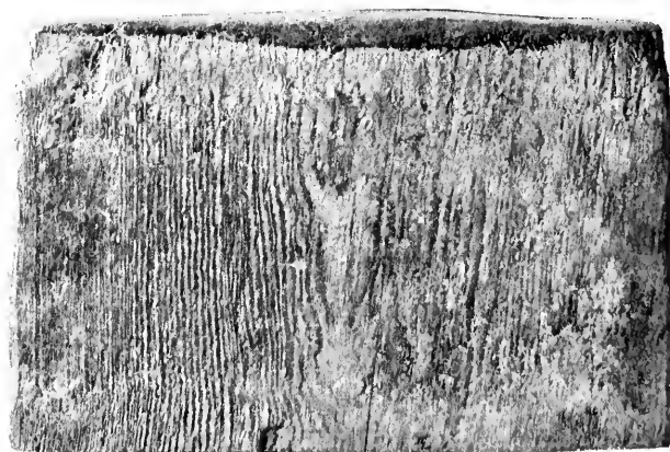
LONG LEAF PINE PAVING BLOCK, AFTER 28 YEARS' USE Laid on Market St., Galveston, in 1875. Removed in 1903. Creosoted.
