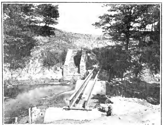
SAME AS ABOVE, DURING CONSTRUCTION
