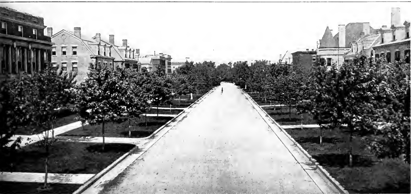
HORTENSE PLACE, ST. LOUIS, SHOWING PROVISION FOR INCREASE OF ROADWAY AND SIDEWALK TRAFFIC
