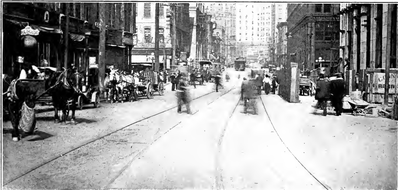
BROAD STREET, LOOKING NORTH FROM VIADUCT
