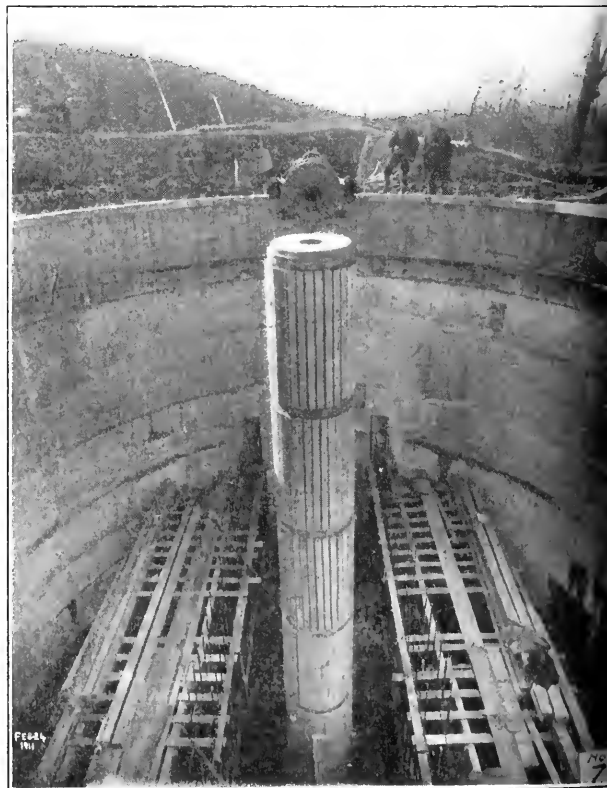
INTERIOR OF PUMP WELL Showing steel reinforcement of partition walls
