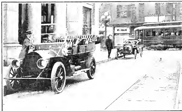
HOUSTON STREET, CANDLER BUILDING ON THE LEFT
