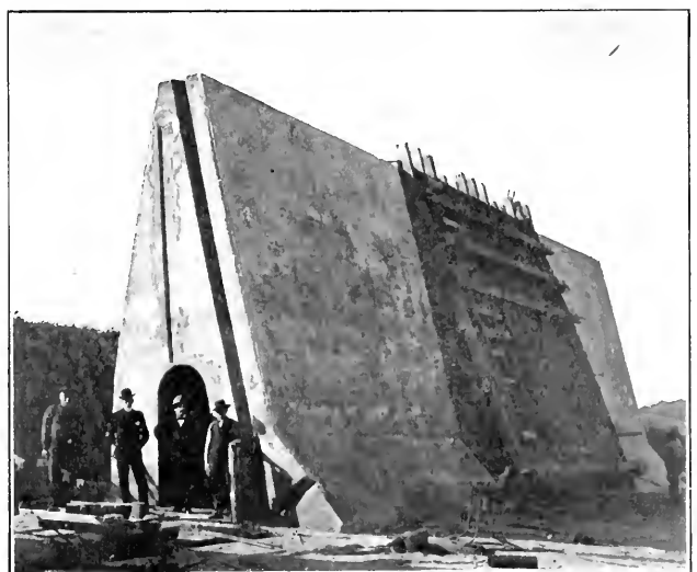
WALL BLOCK, COBB'S HILL RESERVOIR, SHOWING BONDING GROOVE AND KEYWAY
