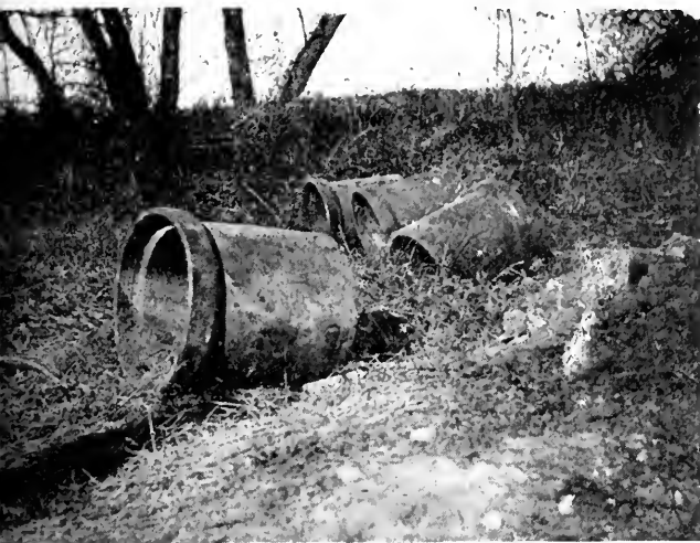
VITRIFIED PIPES READY TO BE LAID FOR CULVERTS
