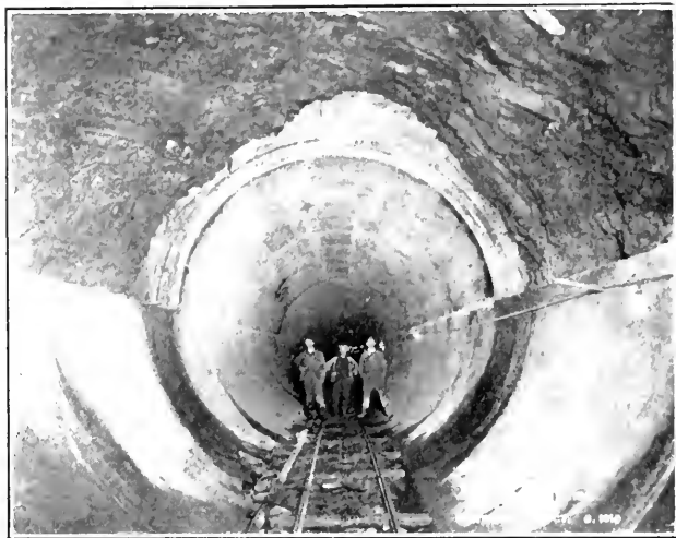
TUNNEL LINING COMPLETED, AND WITH SIDE WALLS ONLY COMPLETED
