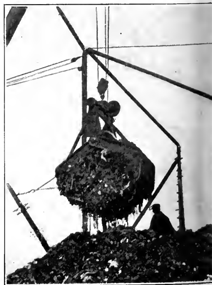
BROWNING AUTOMATIC GRAPPLE LIFTING LOAD OF GARBAGE
