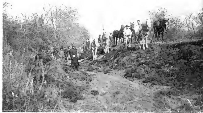
PART OF ROAD AS IT APPEARED IN THE MORNING
