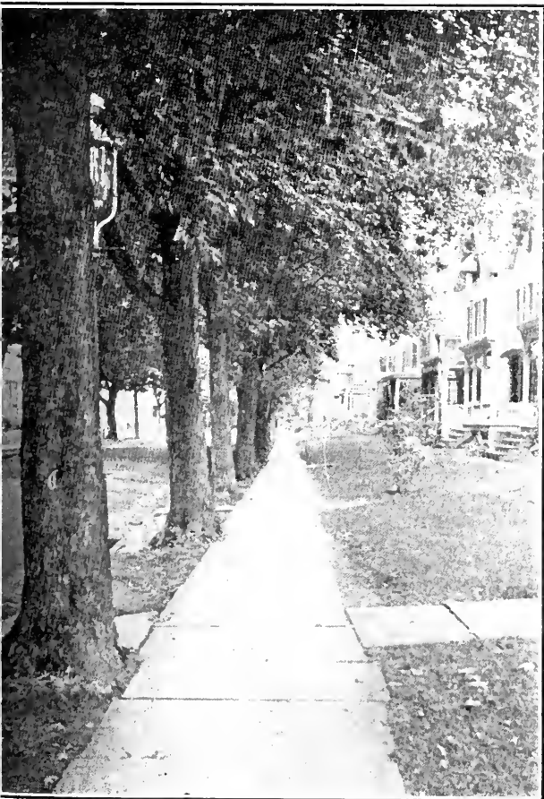
SIDEWALK BEFORE REPAIRING
