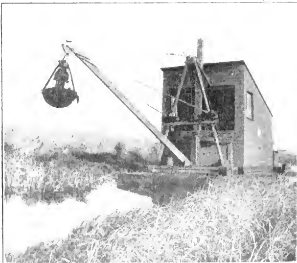
DREDGE AT WORK
