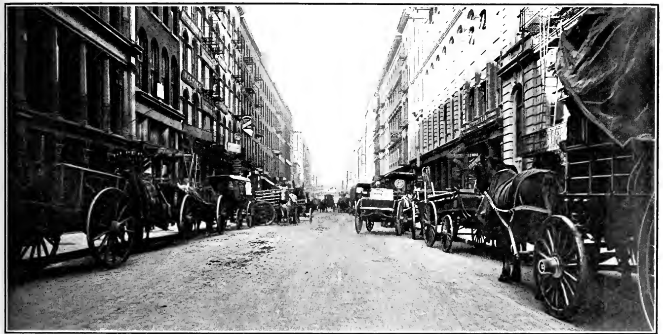
READE STREET, NEW YORK. A TYPICAL WOOD BLOCK PAVED STREET
