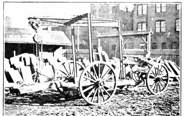
STONE WAGON EQUIPPED WITH ONE-TON HOIST AND TROLLEY
