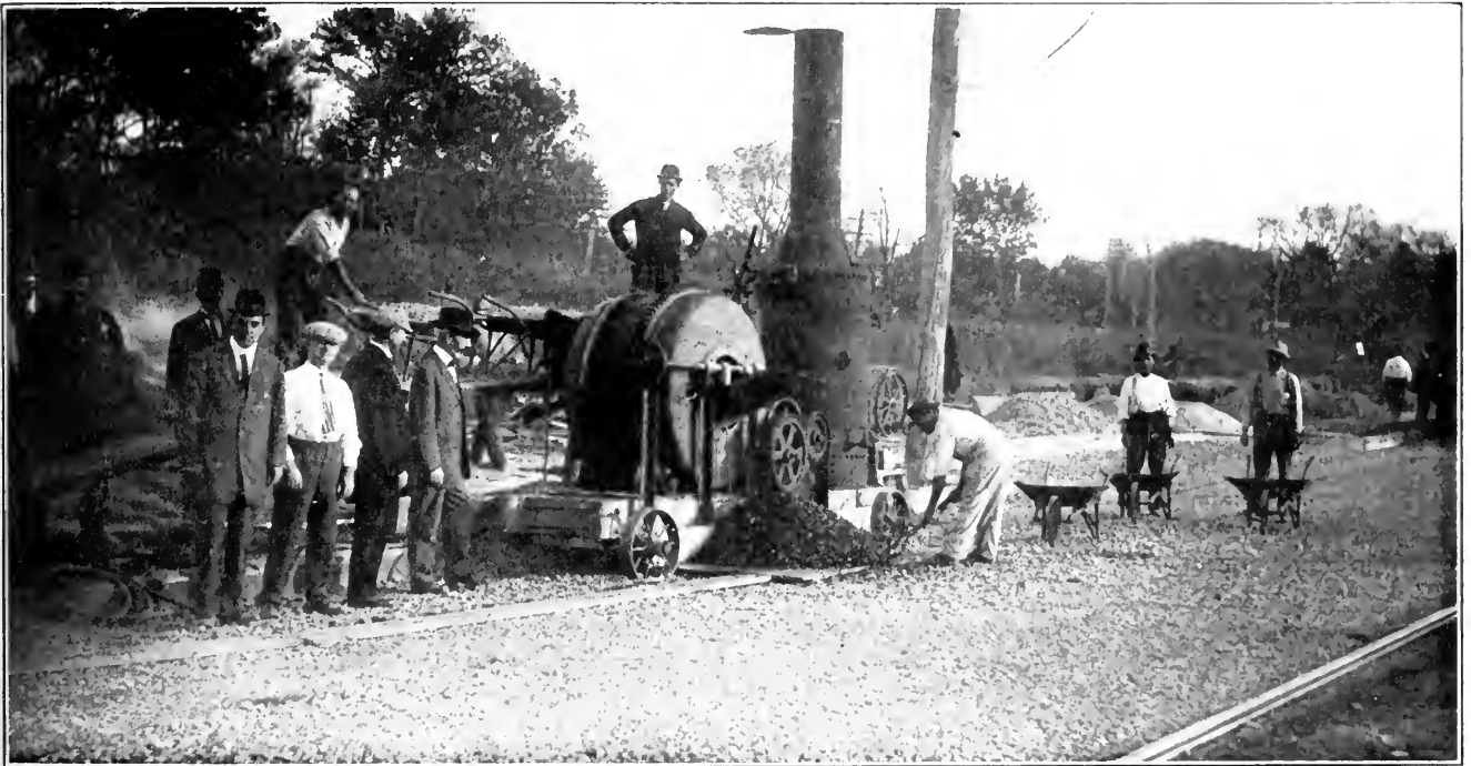
MIXING WITH STANDARD CONCRETE MIXER, SECTION NO. 5
