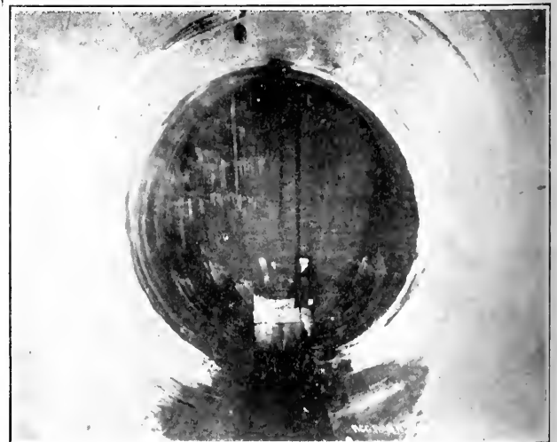
ROUNDOUT SIPHON. LINED TUNNEL SHOWING QUARTER BEND TO UPTAKE SHAFT
