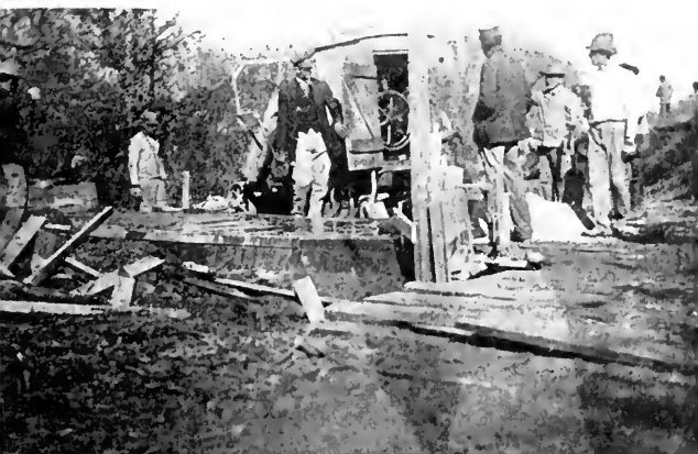
BUILDING CONCRETE BRIDGE CULVERT
