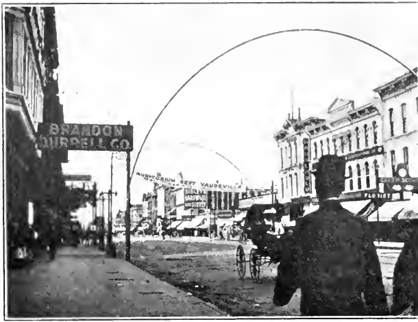
ARCHES IN SOUTH BEND, IND. Appearance in daylight not pleasing
