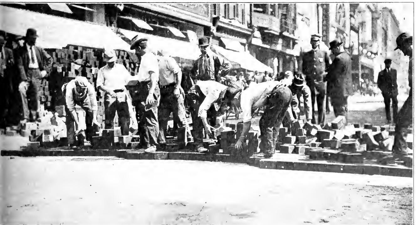
LAYING WOOD BLOCKS ON MARKET STREET NEAR TENTH STREET, PHILADELPHIA
