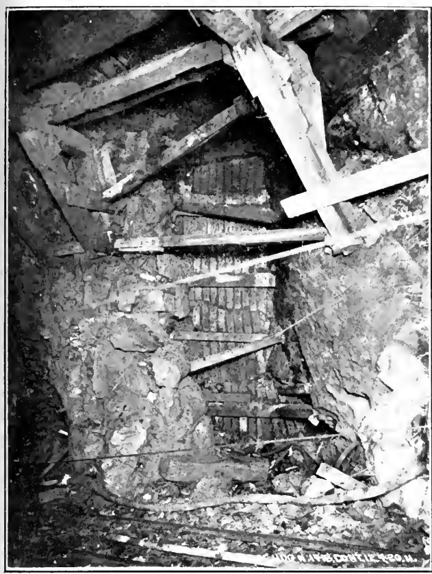
STEEL LAGGING IN MUD SEAM IN SIDE OF TUNNEL
