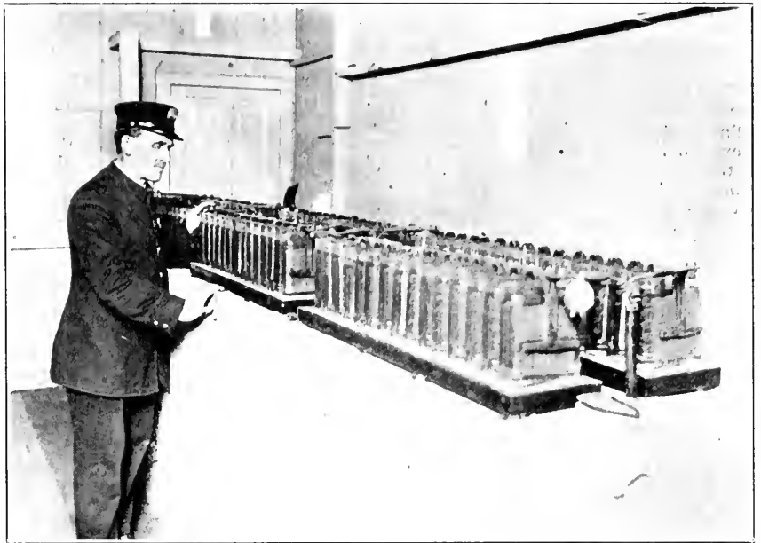
STORAGE BATTERY, SANDUSKY, O., FIRE ALARM SYSTEM
