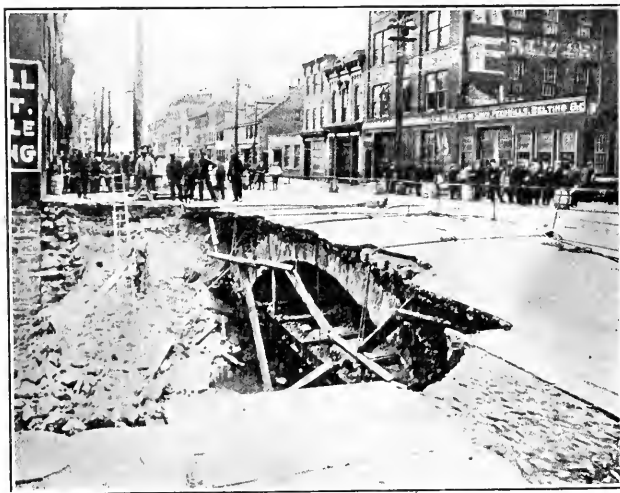
LEAKAGE FROM SEWER BREAKS DOWN OLD BRIDGE
