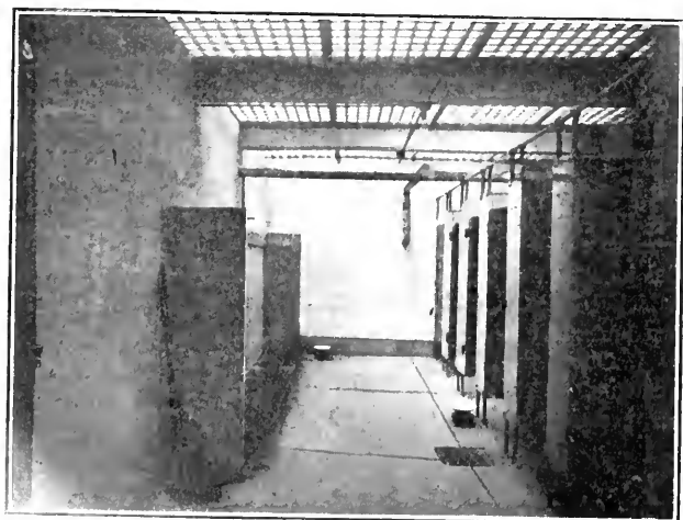
INTERIOR OF MEN'S TOILET ROOM
