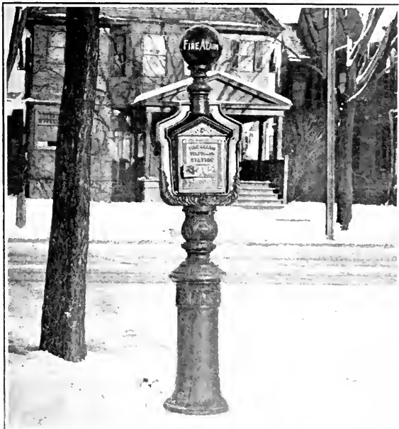
Courtesy Electrical World
