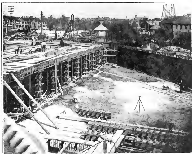
JACKSONVILLE COVERED RESERVOIR UNDER CONSTRUCTION
