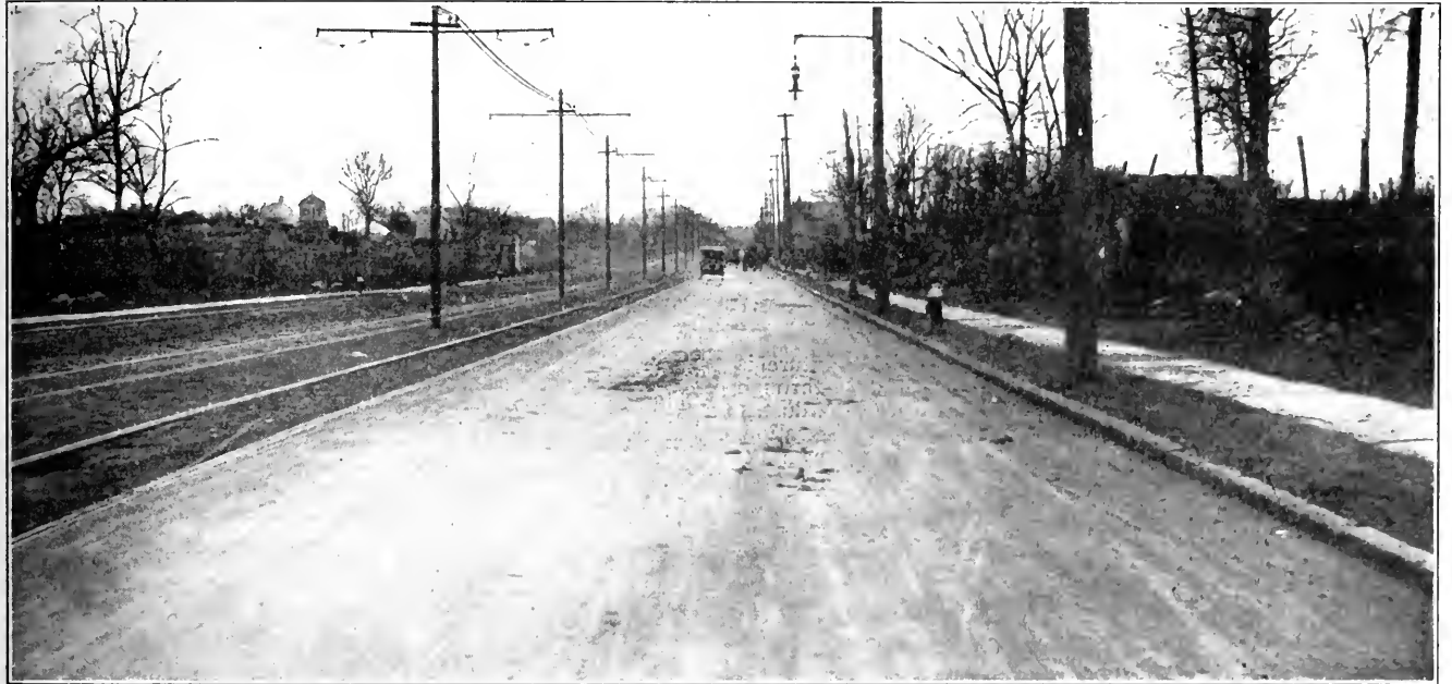
COMPLETED SECTION OF WHITE PLAINS EXPERIMENTAL ROAD Section No. 8 in foreground
