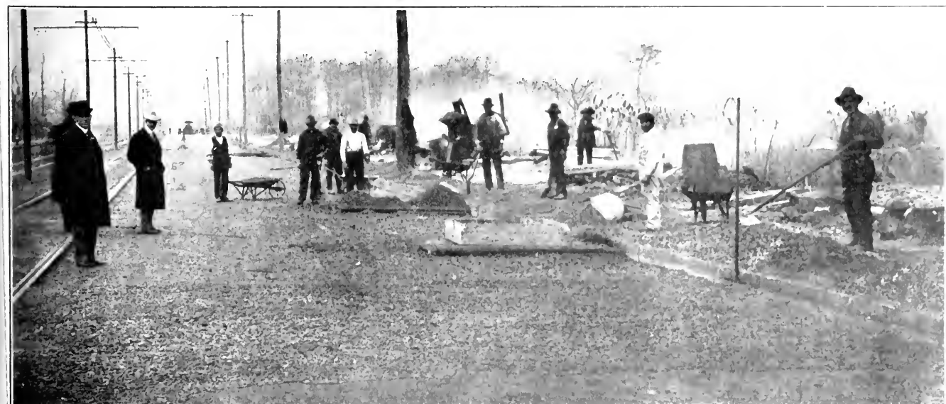
HAND MIXING ON SECTION NO. 4 WHITE PLAINS EXPERIMENTAL ROAD.
