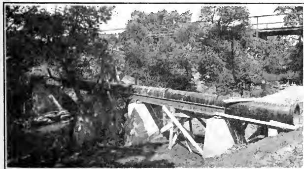
HIGH LEVEL INTERCEPTING SEWER AT CREEK CROSSING
