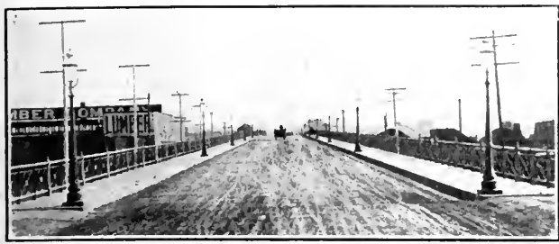
OLD WOODEN VIADUCT, NOW BEING TAKEN DOWN
