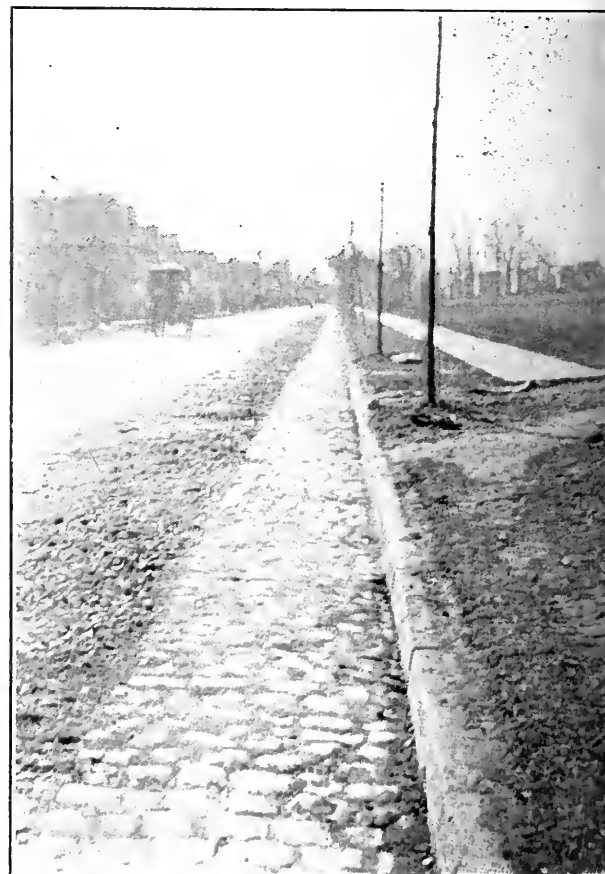
CURB AND GUTTER AFTER REPAIRING
