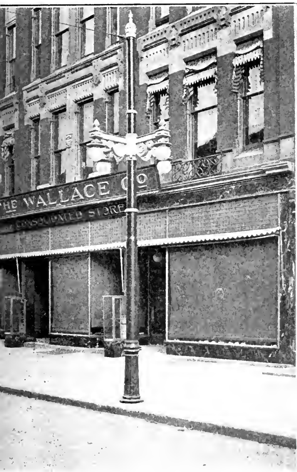
STANDARD LAMP AND TROLLEY POLE
