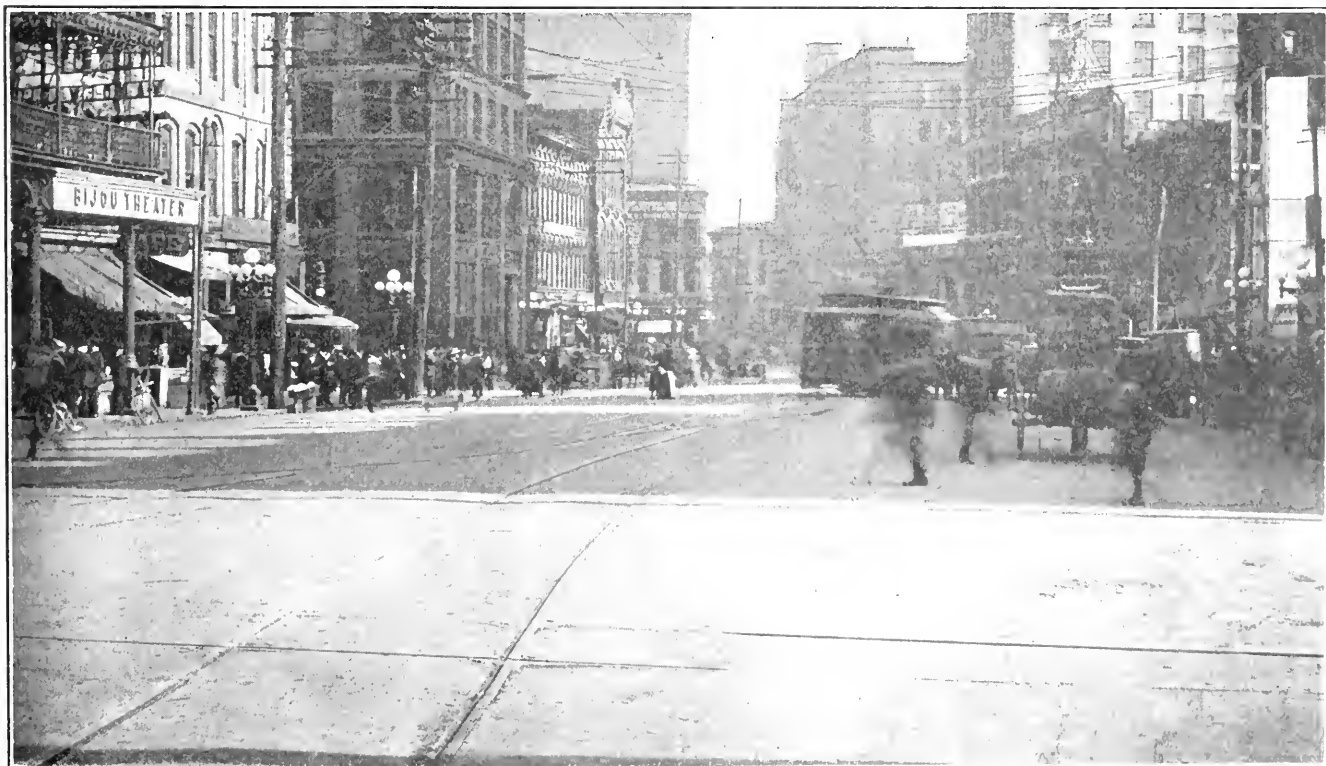
MARIETTA STREET AT INTERSECTION WITH NORTH FORSYTH STREET
