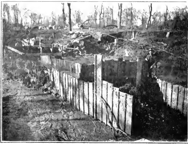
WHERE RIVER BROKE INTO TRENCH.
