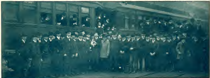
ON THE INSPECTION TOUR
