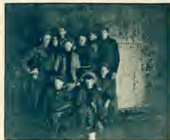
'04's as Tank Painters
