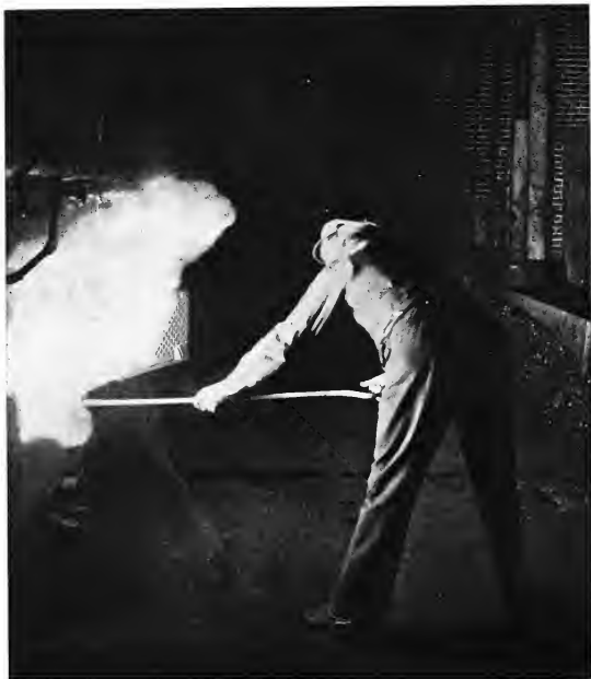
THE OLD BOILER ROOM—THE LAST FIRE
