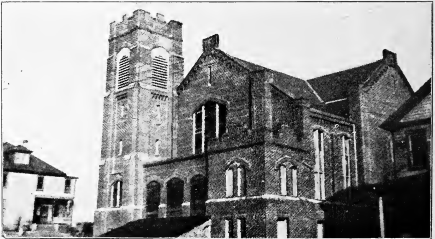
Second U. B. Church, Martinsburg, W. Va.—Not yet Completed. Cost, $40,000
