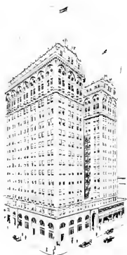
Jefferson Standard Building
