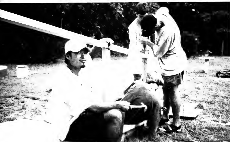
Some members of HOME hard at work on a fine spring day.
