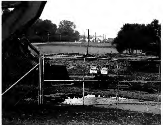
The construction of the Frank Family Science Center begins.
