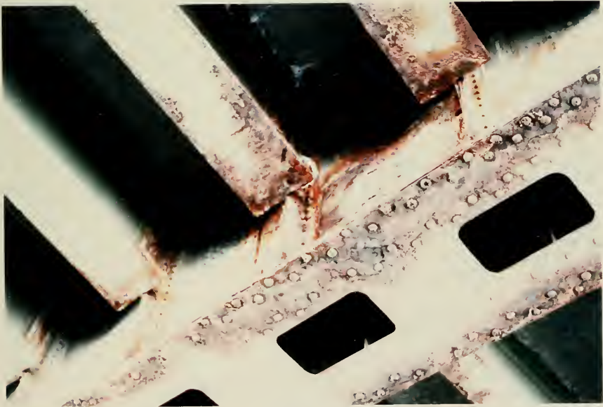
Sullivan Square Rehabilitation Charlestown, Massachusetts
