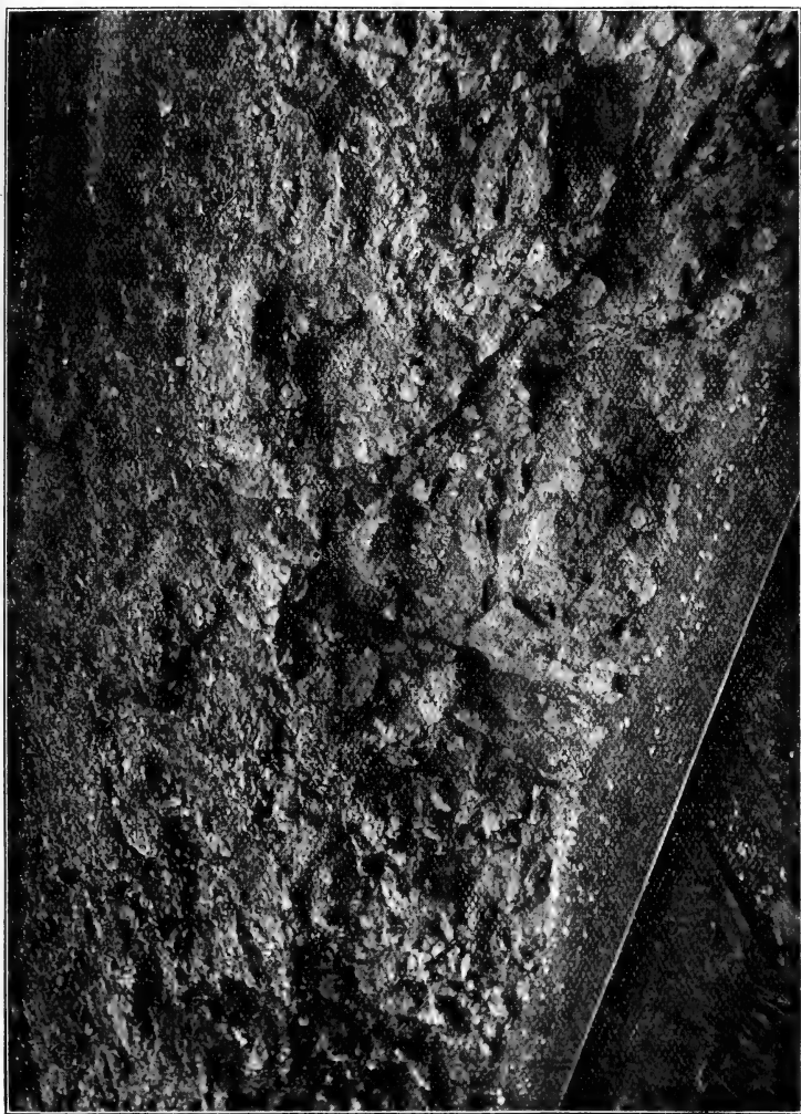
Fig. 4.—Another part of the same railway-cutting as that seen in fig. 3, showing a second fold in the beds of white knoll limestone.
