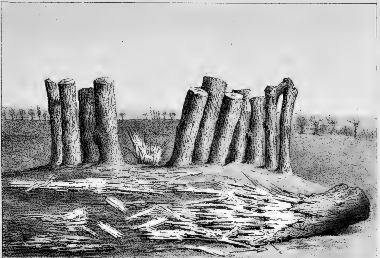
EXPLOSIVE EFFECTS OF THE FIRST CHARGE OF ENGLISH MADE GUN COTTON ( Two views of the Stockade )
