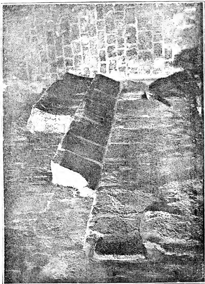
[From a Photograph by G. R. Leco.] SPRING OF ARCH IN "SOLOMON'S STABLES," RECENTLY DISCOVERED.
