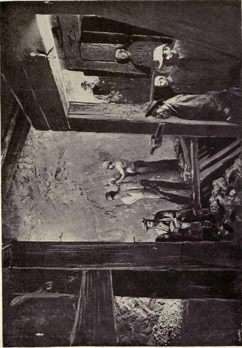
STOPE OR "LABORE," NEW ALMADEN QUICKSILVER MINE.
