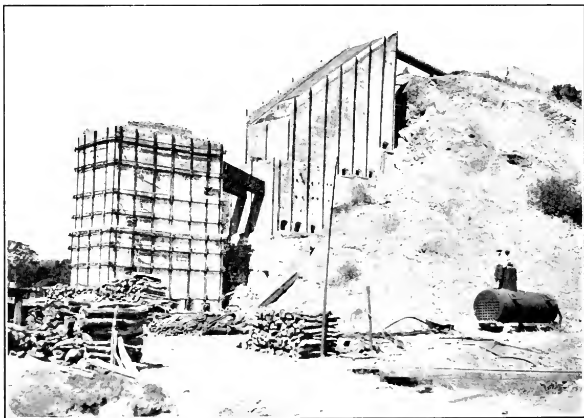
Photo No. 56. Scott Furnace and Condensers at Klau Mine, San Luis Obispo County. Sloping top of condenser chambers was covered with sheet-iron and used as an ore drier. The enclosing building was destroyed by fire a few years ago.
