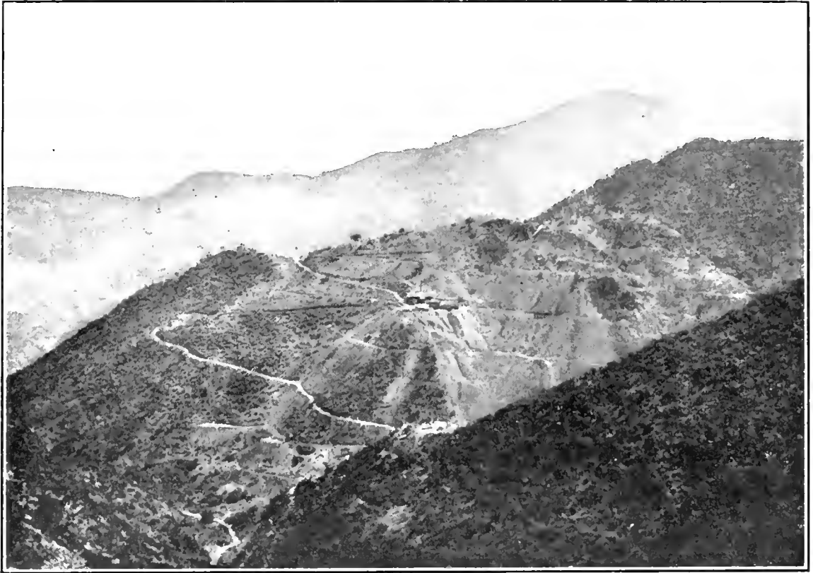
Photo No. 24. New Idria Mine, showing open cuts and dumps being reworked at top of hill. Much of this is to be quarried off. Buildings in center are at portal of No. 2 level.
