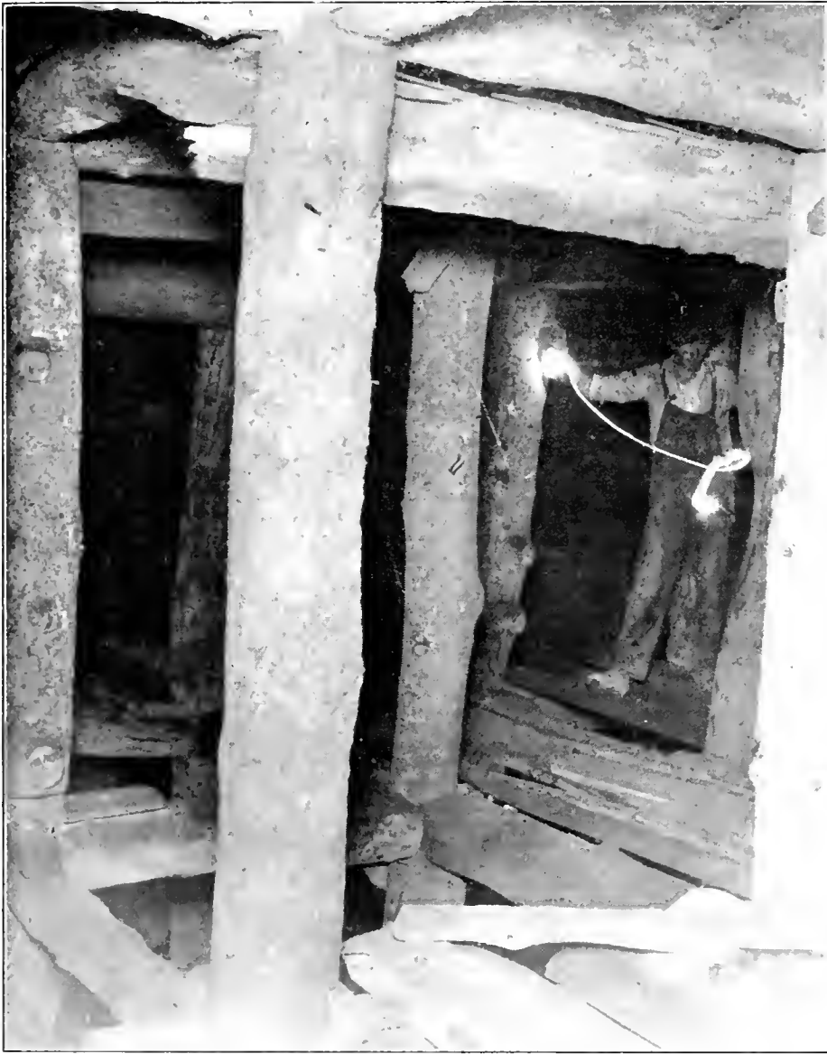
Photo No. 22. Flashlight view in square set stope (30' wide) between No. 2 and No. 2 \frac{1}{2} levels, New Idria Mine.
