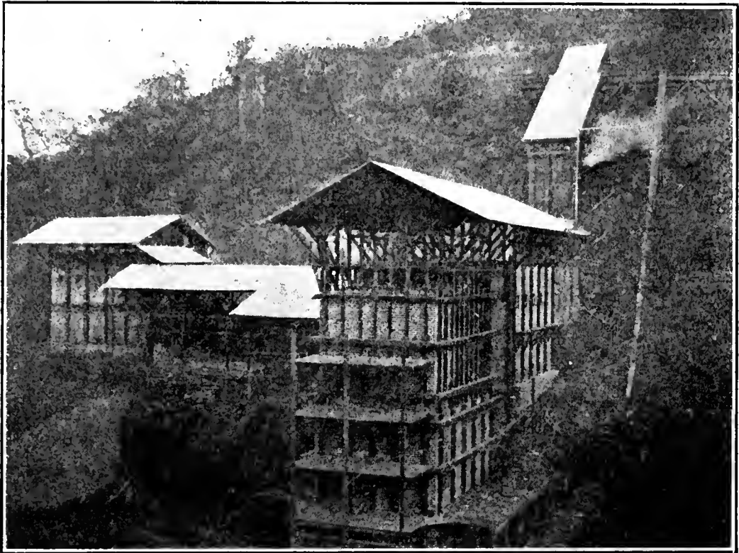
Photo No. 40. Fifty-ton Scott furnace and condensers at Phoenix Mines, Stanislaus County. Photo by F. L. Lowell.
