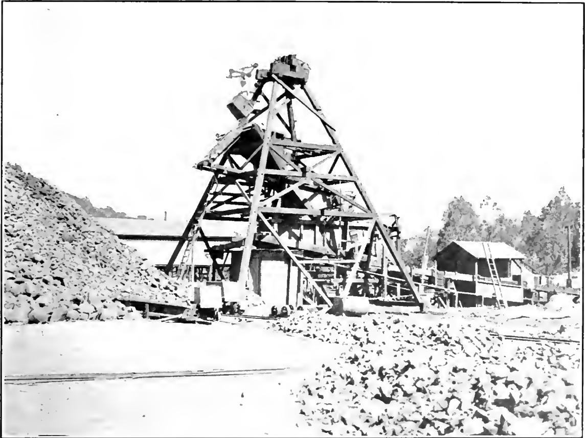
Photo No. 77. Gravel-washing plant for recovering metallic quicksilver from material excavated from old furnace sites, at Hacienda of New Almaden Company, Santa Clara County.
