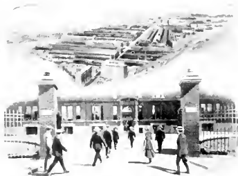
MAIN PLANT GENERAL ELECTRIC COMPANY
