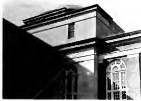
CHAMBERS BUILDING FROM THE REAR
