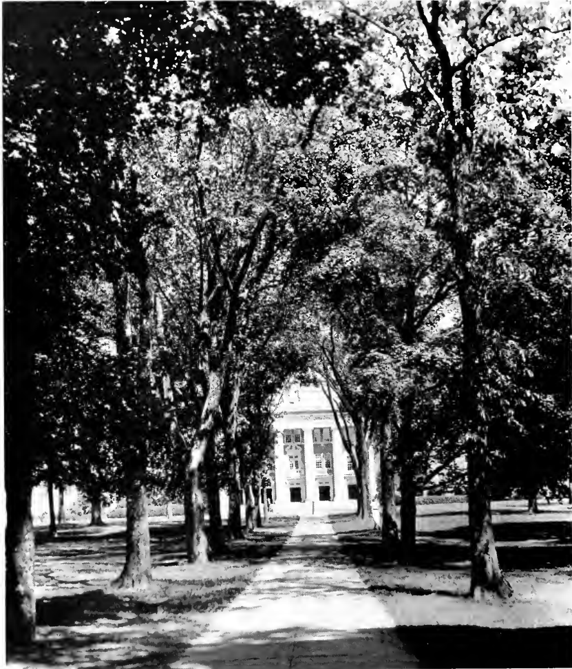
FRONT WALK TO CHAMBERS BUILDING
